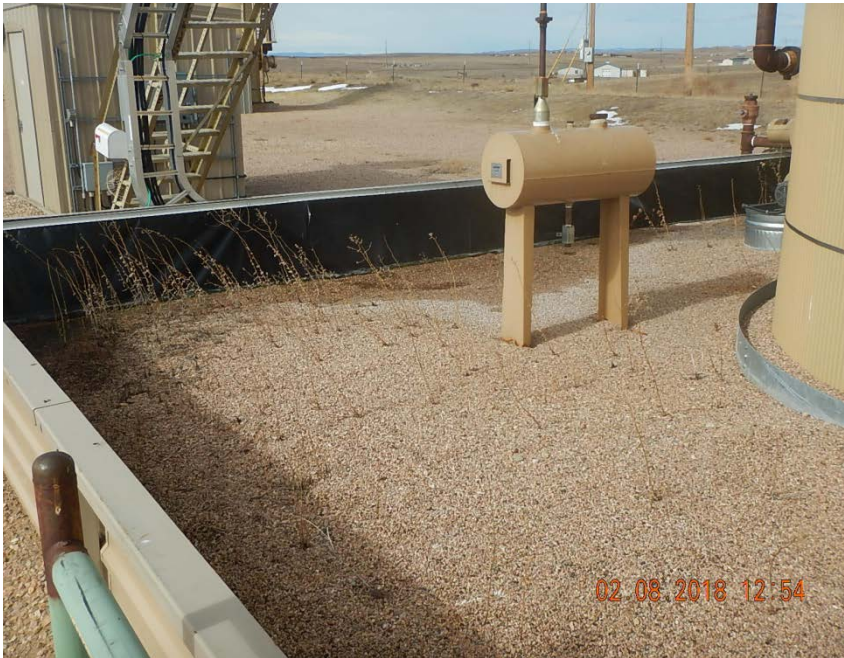
Photo 9: Weeds in tank battery berm
