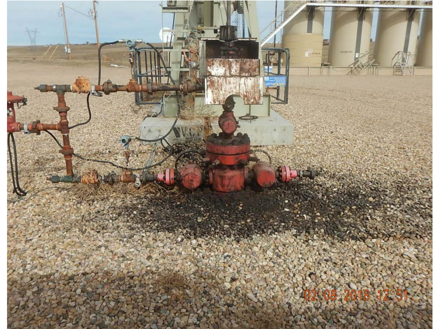
Photo 2: Wellhead, looking N. Stained soil around wellhead.
