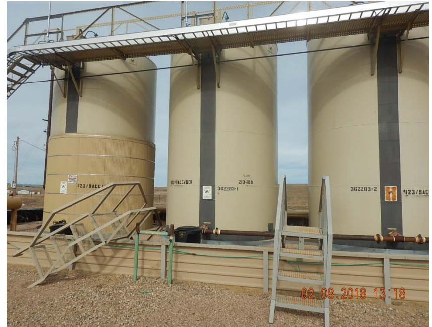
Photo 10: Tanks not labeled with capacities
