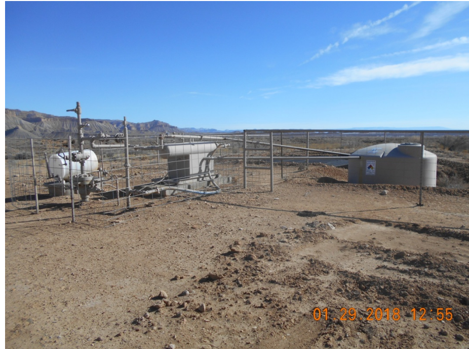
Wellhead with chemical drum with secondary containment. Separator and tank
