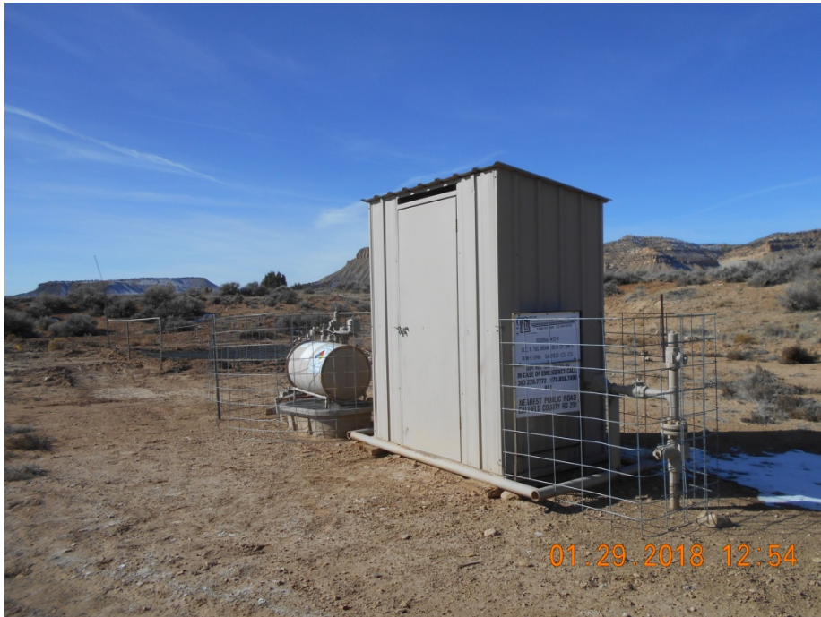
Meter housing and chemical drum with secondary containment.
