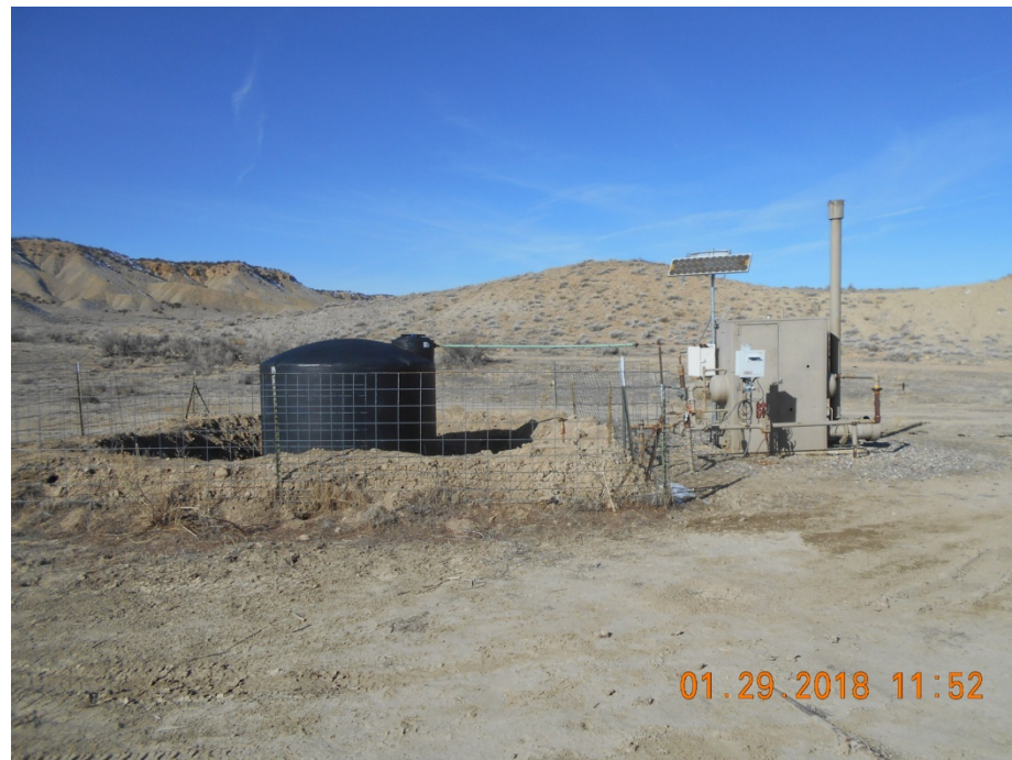
Separator and tank battery.
