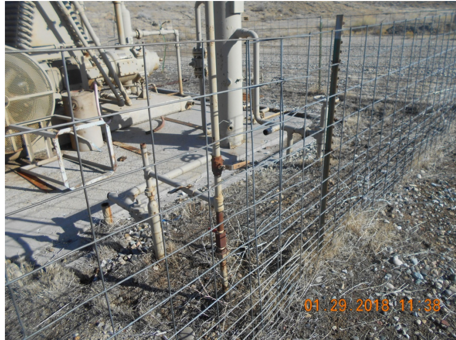
Unused unmarked risers at compressor.
