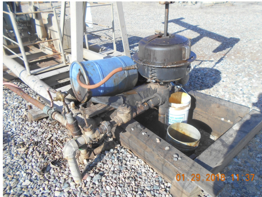
Stained soil at wellhead and improper handling of E&P waste.
