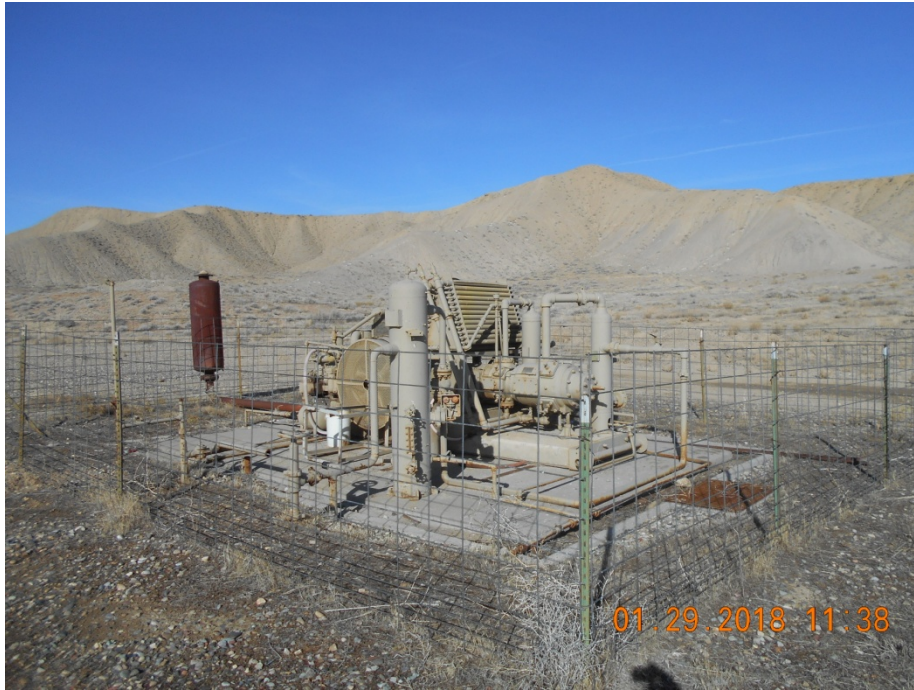
Compressor with unused/unmarked risers.
