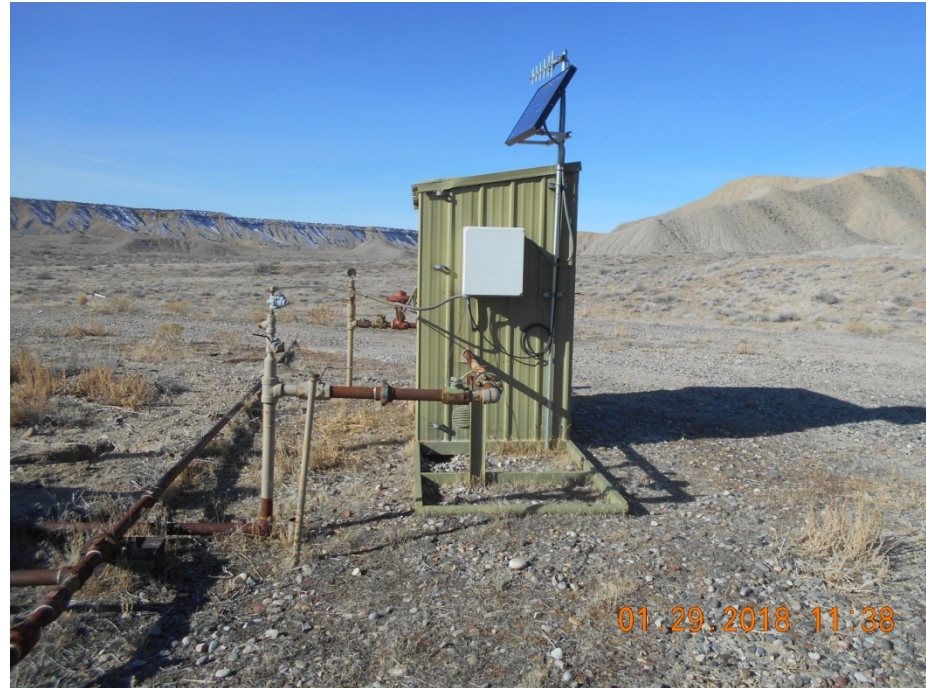
Meter house with unused/unmarked risers.
