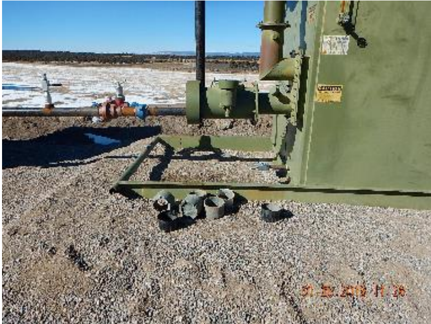
Photo 7: Thread protectors at separator.
