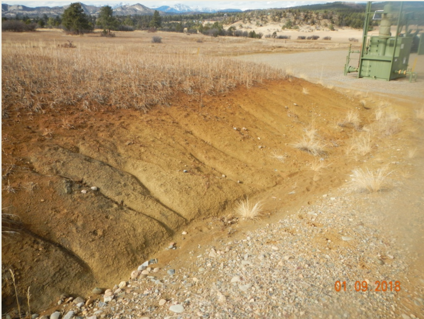
Photo 6. View of erosion occurring along the western portion of the access road.
