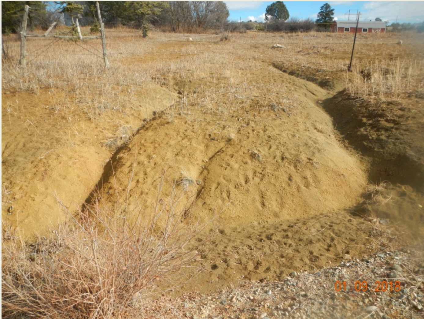
Photo 5. View of erosion along the eastern edge of the access road.
