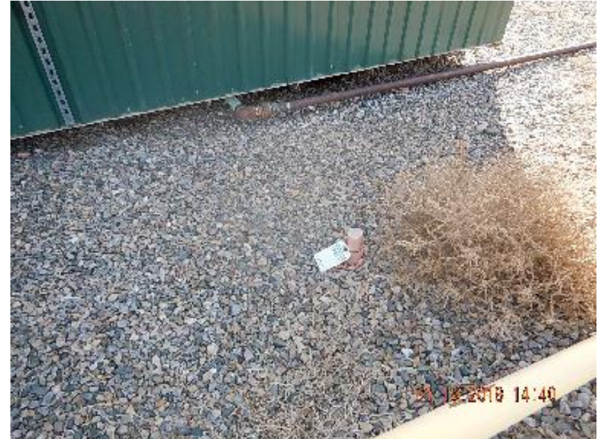
Photo 8: Painted, plugged, and tagged 2" riser outside pump building.
