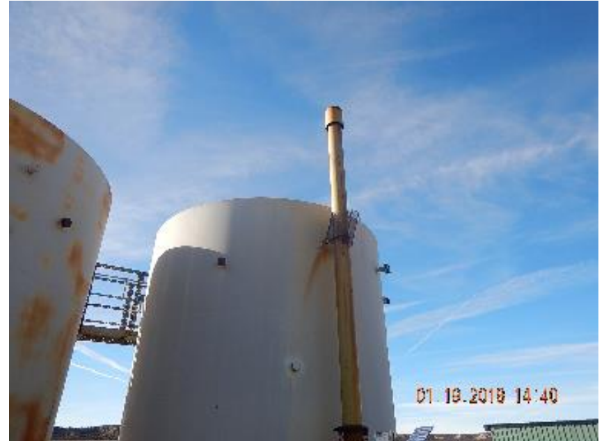
Photo 10: Wildlife protection screen slid down stack.
