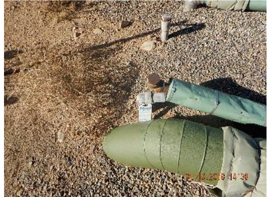
Photo 6: (2) painted, plugged, and tagged 2" risers behind storage building.
