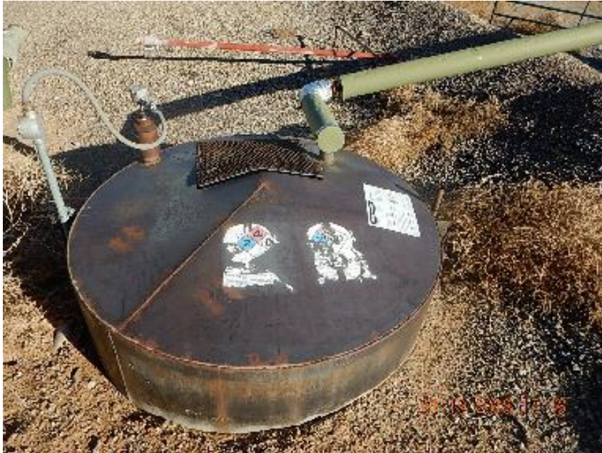
Photo 13: Peeling labels on 21 BBL tank.
