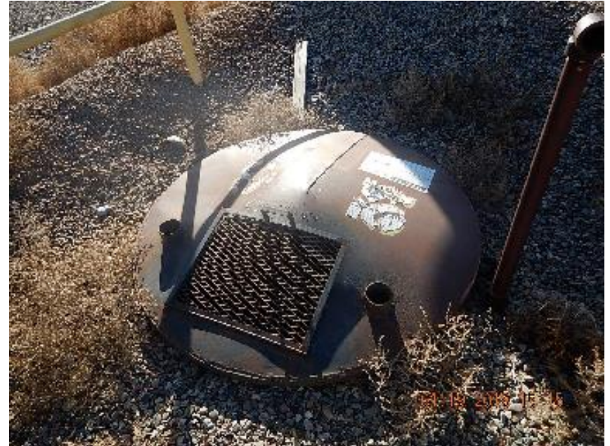
Photo 14: Peeling labels on 21 BBL tank.
