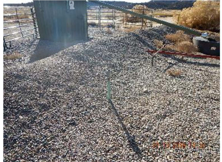
Photo 4: (2) 1" risers out from small equipment building and 21 BBL tank.
