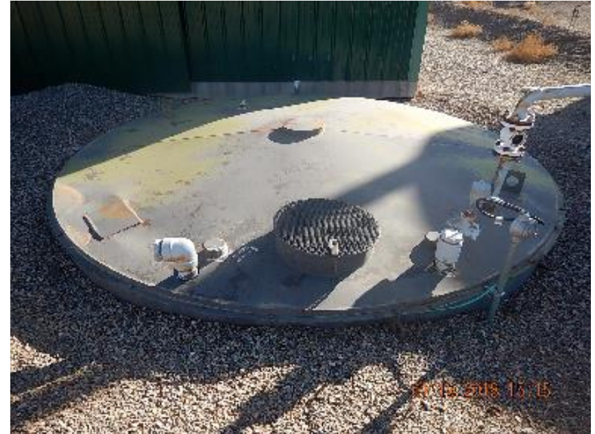
Photo 12: 95 BBL tank with no labels or signage.
