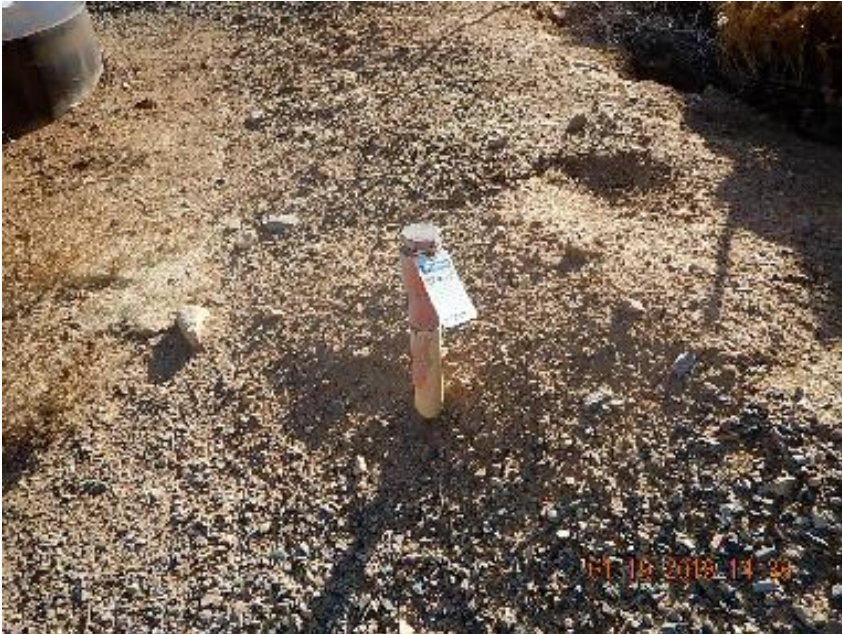
Photo 7: Painted, plugged, and tagged 2" riser behind storage building and at rear berm.
