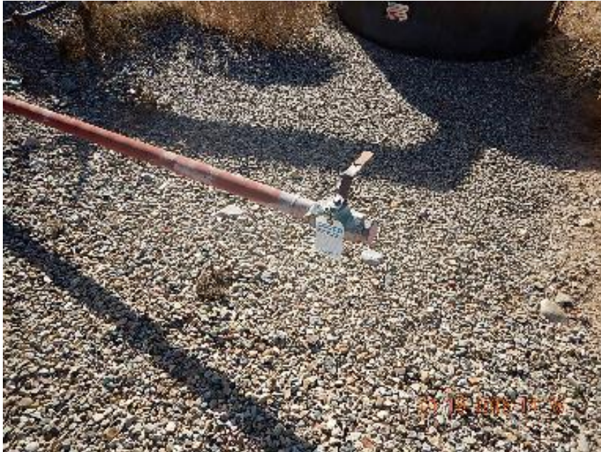
Photo 5: Painted, plugged, and tagged 2" line out from small equipment building and 21 BBL tank.
