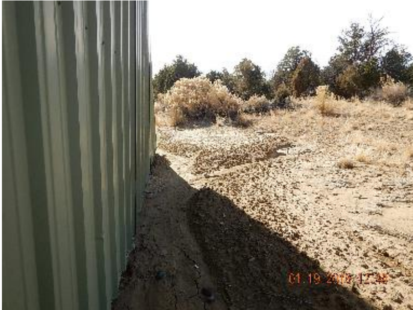
Photo 5: Erosion channel on backside of compressor sound wall.
