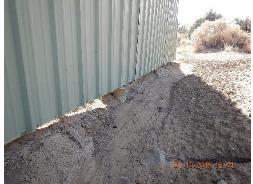
Photo 6: Erosion around wall concrete footings.
