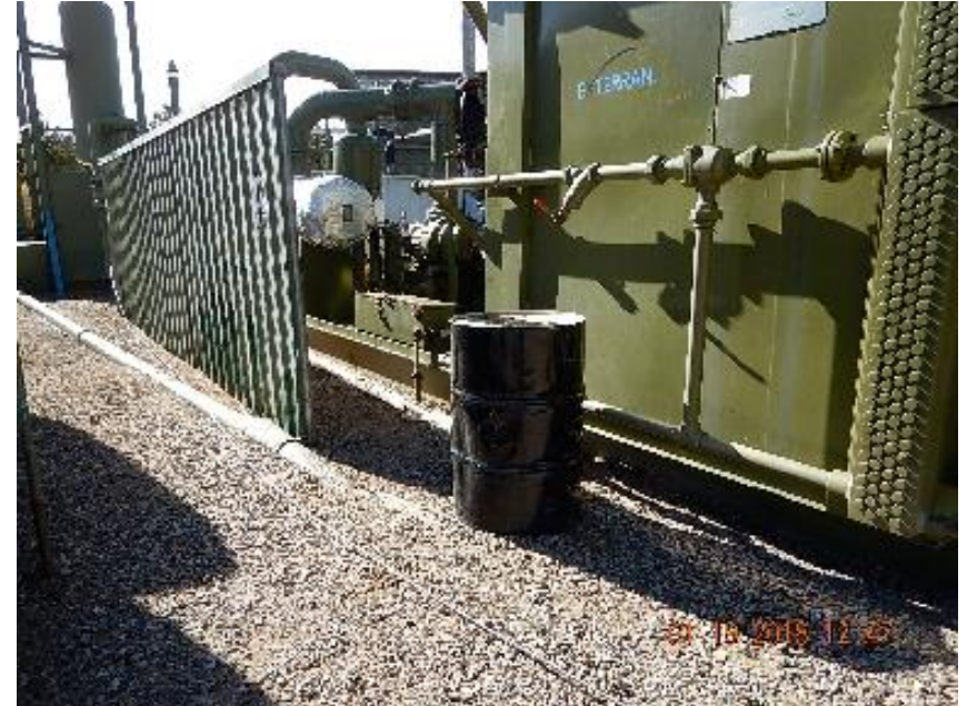
Photo 4: 55 gallon drum without spill prevention.
