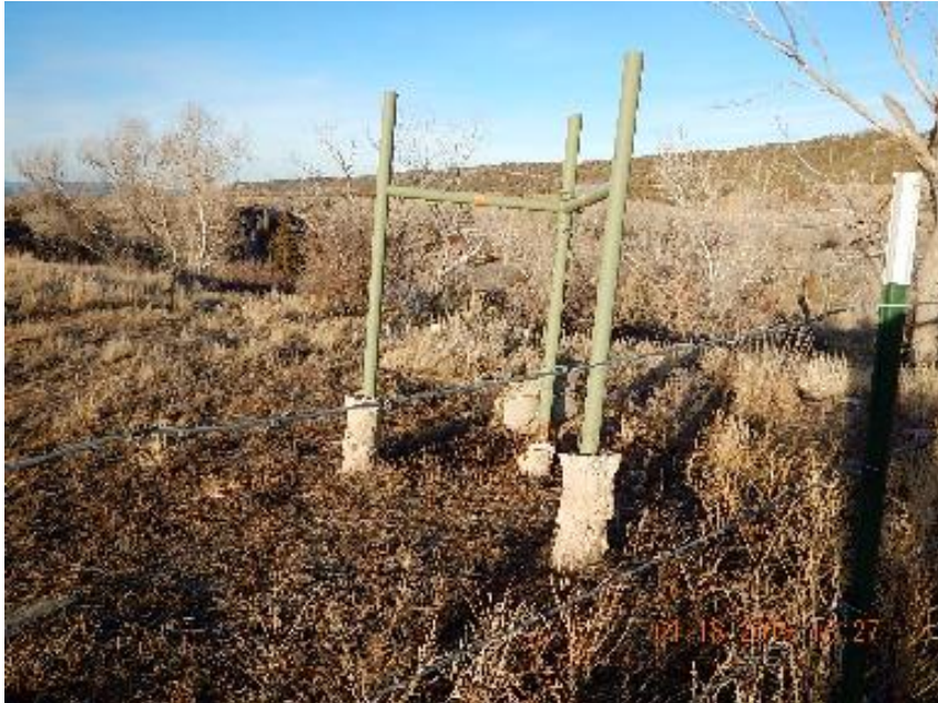
Photo 5: Fence corner brace in NE corner.
