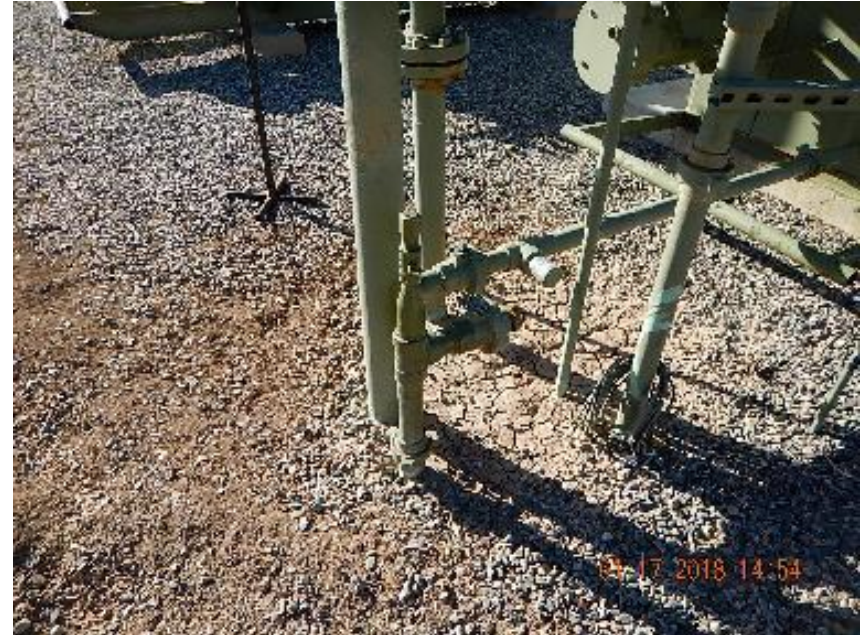
Photo 4: Unused riser at separator.
