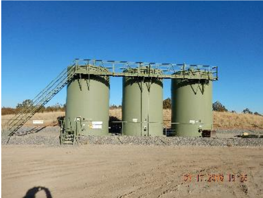
Photo 5: Tank battery with no visible NFPA label.
