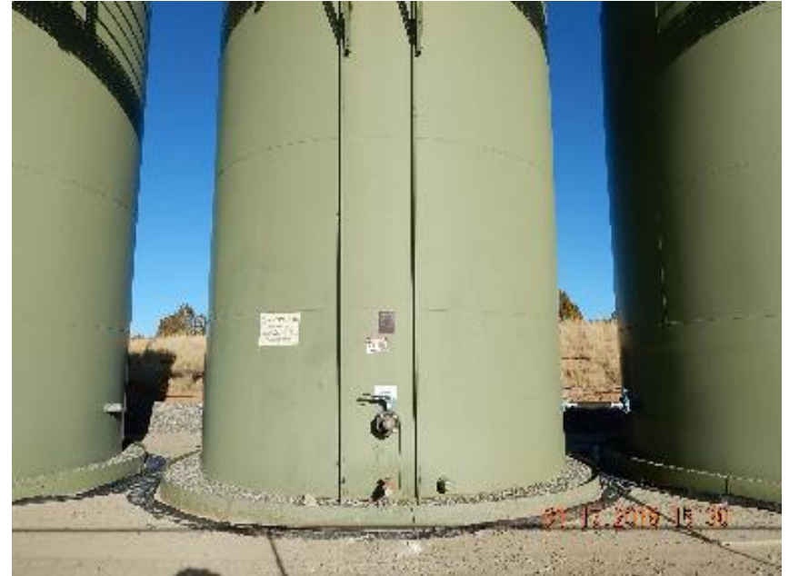
Photo 6: Closer view on tank labels. Black label above valve is unreadable NFPA label.
