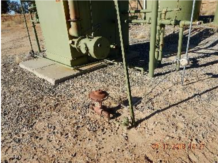
Photo 3: 1" unused steel riser at separator. Valve plugged but not tagged.
