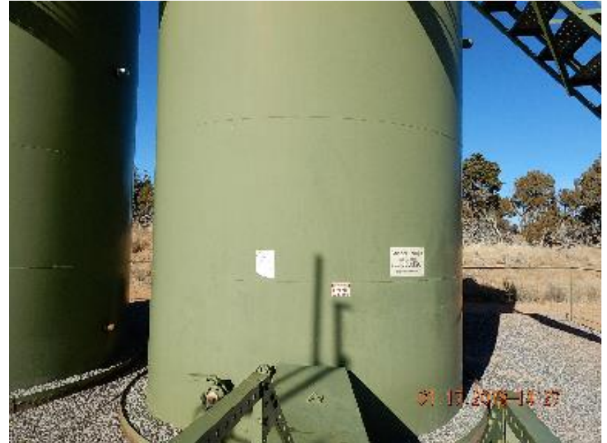
Photo 2: 500 BBL tank without NFPA label.
