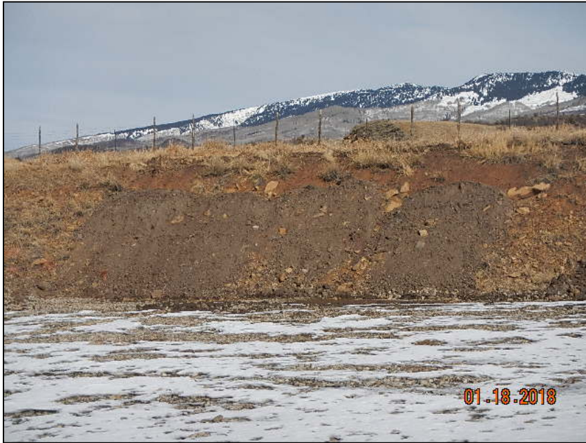
Photo 1. Top soil has been placed on cut slope to mitigate erosion. Site will need to be reevaluated in the future. Tanks have been removed from location.
