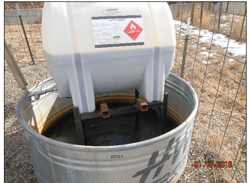
Photo 4. Tank photo from current inspection. Chemical is present in chemical containment at the well head. No cover is in place over containment, and is open to wildlife.
