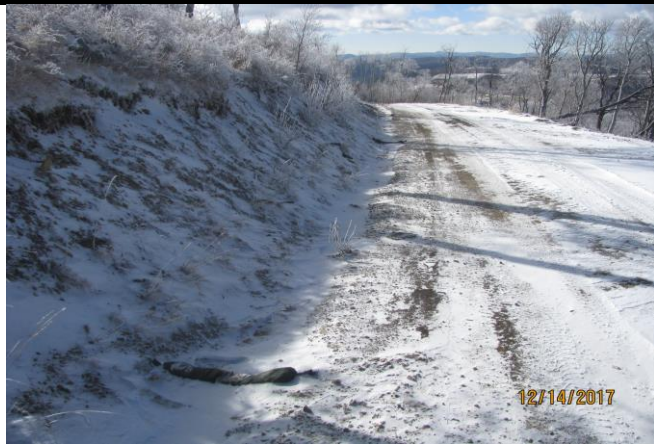
Rock Sock Installation on the C.C. 610-24-43 Access Road
