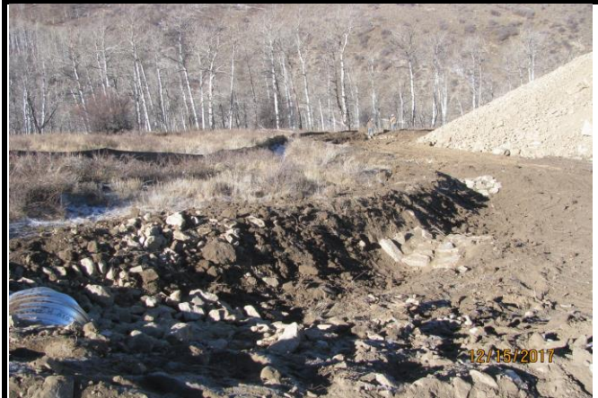
Dewatering Channel and Rock Checks in the SW Corner of the C.C. 697-03-07 Pad
