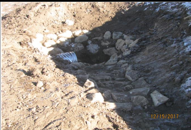
Rock Armor Installation on Culvert Inlet on the C.C. 697-03-07 Access Road
