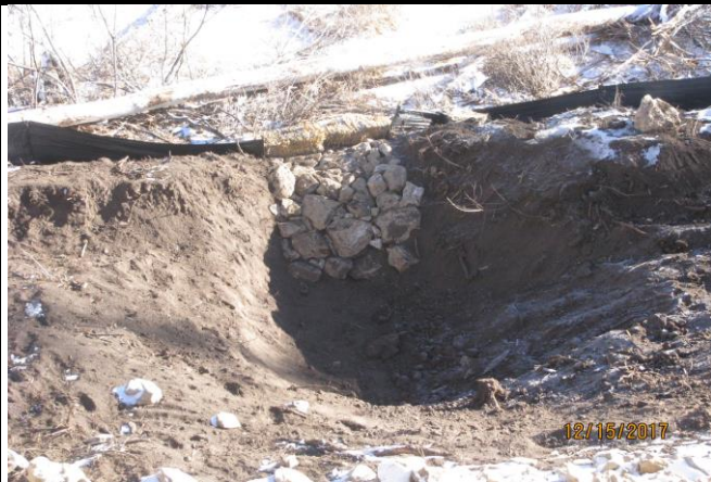
Rock Apron Outlet Installation on the East Side of the C.C. 697-03-07 Pad
