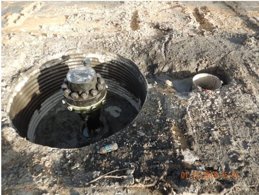
Photo 1. Photo taken from one of the wellheads at location. Photo illustrates a rat hole left open. This is a potential safety and wildlife hazard. Operator should also consider placing safety fence around the wellhead area for safety measures.
