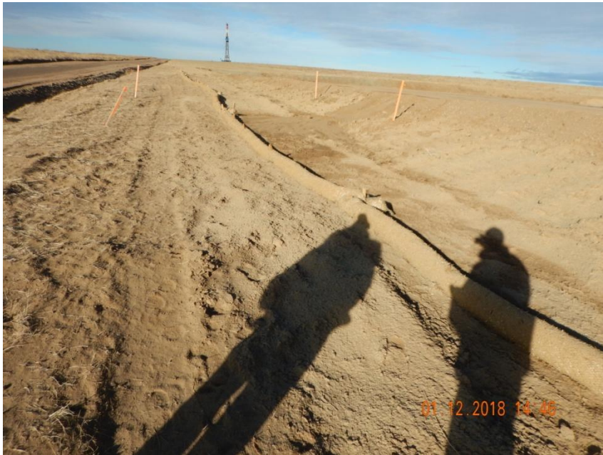
Photo 5. Photo taken from the western perimeter of the location, facing North. Straw wattle BMP has been installed and hydromulch has been applied to unconsolidated soil material along the perimeter of the location.
