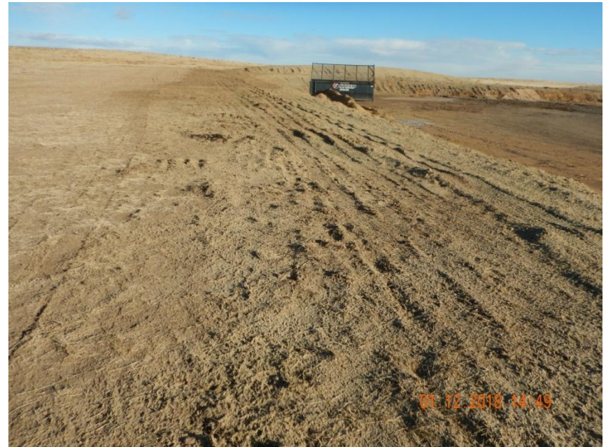
Photo 6. Photo taken from the northern perimeter of the location, facing East. Appears a surface roughening BMP has been installed along portions of the perimeter; however, this does not appear to be a sufficient and appropriate BMP for the sandy soil conditions. Hydromulch has been applied to unconsolidated soil material along the perimeter of the location.
