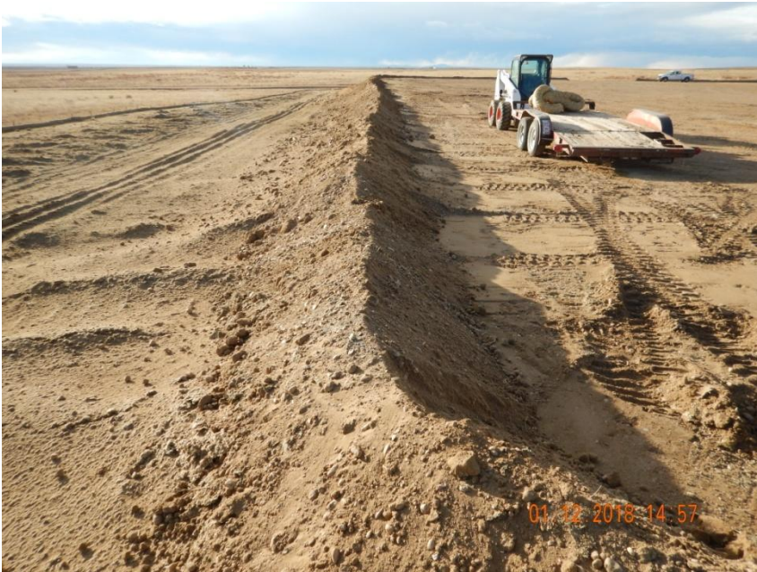
Photo 9. Photo taken from the southeastern perimeter of the location, facing West. Operator has not properly stabilized the berm BMP.
