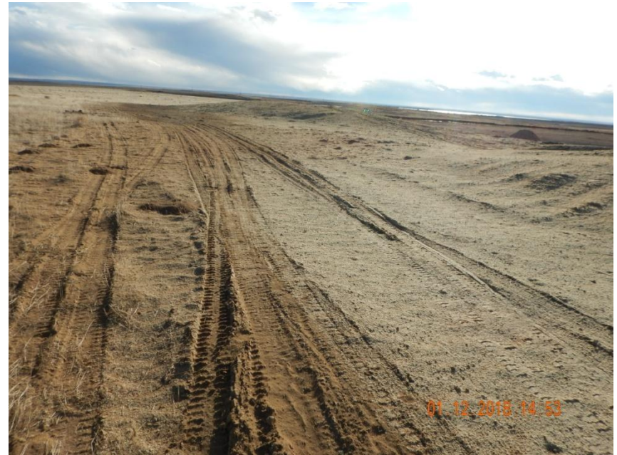
Photo 8. Photo taken from the eastern perimeter of the location, facing South. Appears the Operator has temporarily stabilized the topsoil stockpile with hydromulch. Operator does not have sufficient stormwater BMPs along the perimeter of the location.
