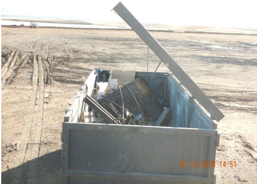
Photo 7. Photo taken from the northern location, facing South. Operator shall keep the trash lid closed to prevent trash from blowing out of containment.
