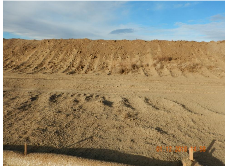
Photo 10. Photo taken from the southern perimeter of the location, facing North. Operator has not sufficiently stabilized the southern fill slope.
