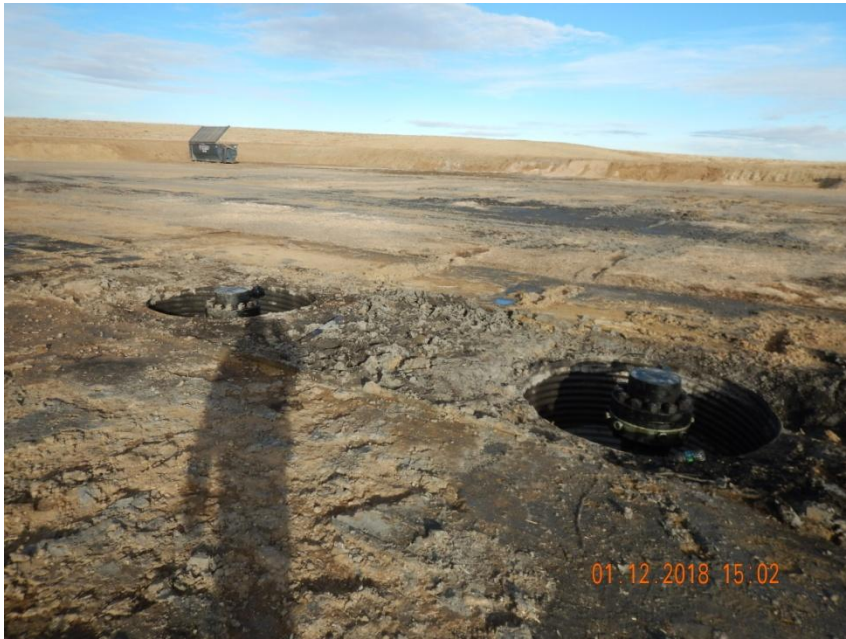
Photo 3. Photo taken from the wellhead area, facing East. Operator has left drill cuttings at location and has not properly transported the drill cuttings off location.
