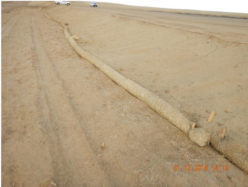
Photo 11. Photo taken from the western perimeter of the location, facing North. Straw wattle BMP has been installed but unconsolidated soil material along the perimeter of the location has not been stabilized.
