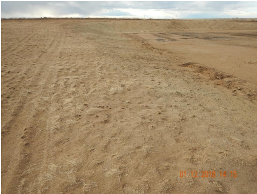
Photo 9. Photo taken from the southern perimeter of the location, facing West. Operator does not have sufficient stormwater BMPs to control stormwater run-on onto location.
