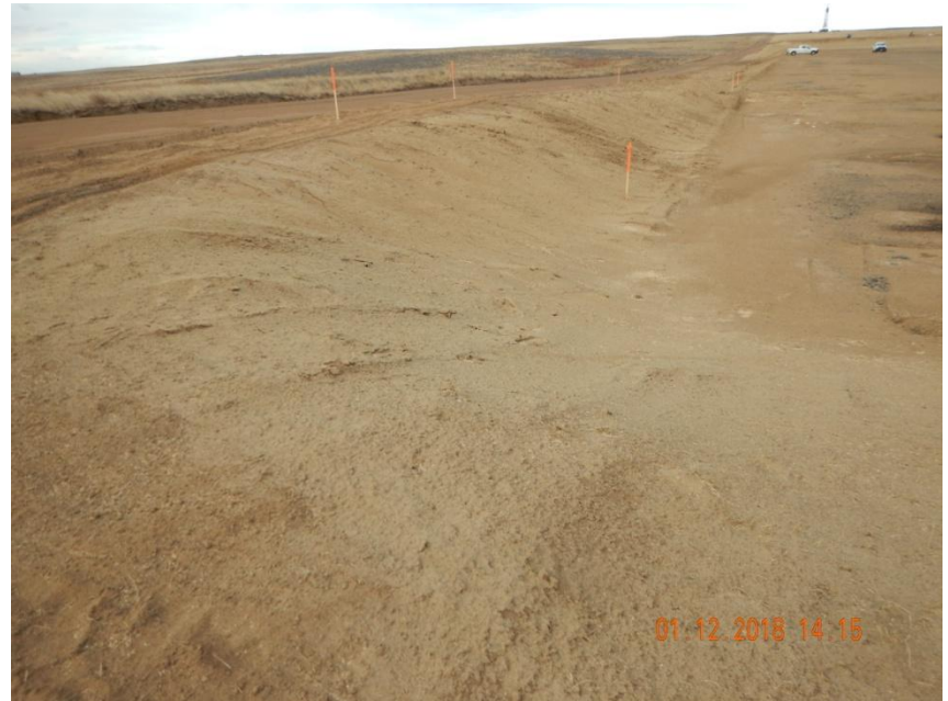
Photo 10. Photo taken from the southwest perimeter of the location, facing North. Operator has applied a hydromulch to the cut slopes as a temporary stabilization BMP.
