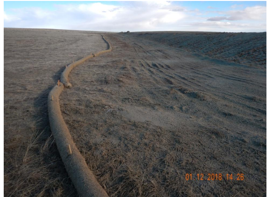
Photo 12. Photo taken from the northwest perimeter of the location, facing East. Straw wattle BMP has been installed and appears hydromulch has been applied to unconsolidated soil material along the perimeter of the location.
