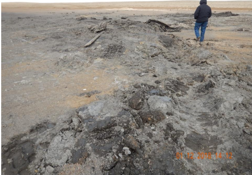
Photo 3. Photo taken from the southern well pad, facing East. Operator has left drill cuttings at location and has not properly transported the drill cuttings off location.
