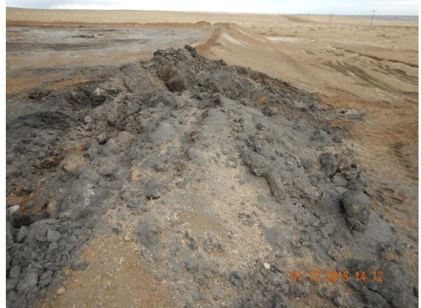
Photo 4. Photo taken from the southern well pad, facing East. Operator has not properly transported and handled drill cuttings at location. Drill cuttings were observed along portions of the fill slope.
