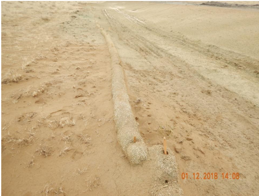
Photo 7. Photo taken from the eastern perimeter of the location, facing South. Appears the Operator has temporarily stabilized the topsoil stockpile with hydromulch. Straw wattle BMP has been installed to the outer perimeter of the stockpile.
