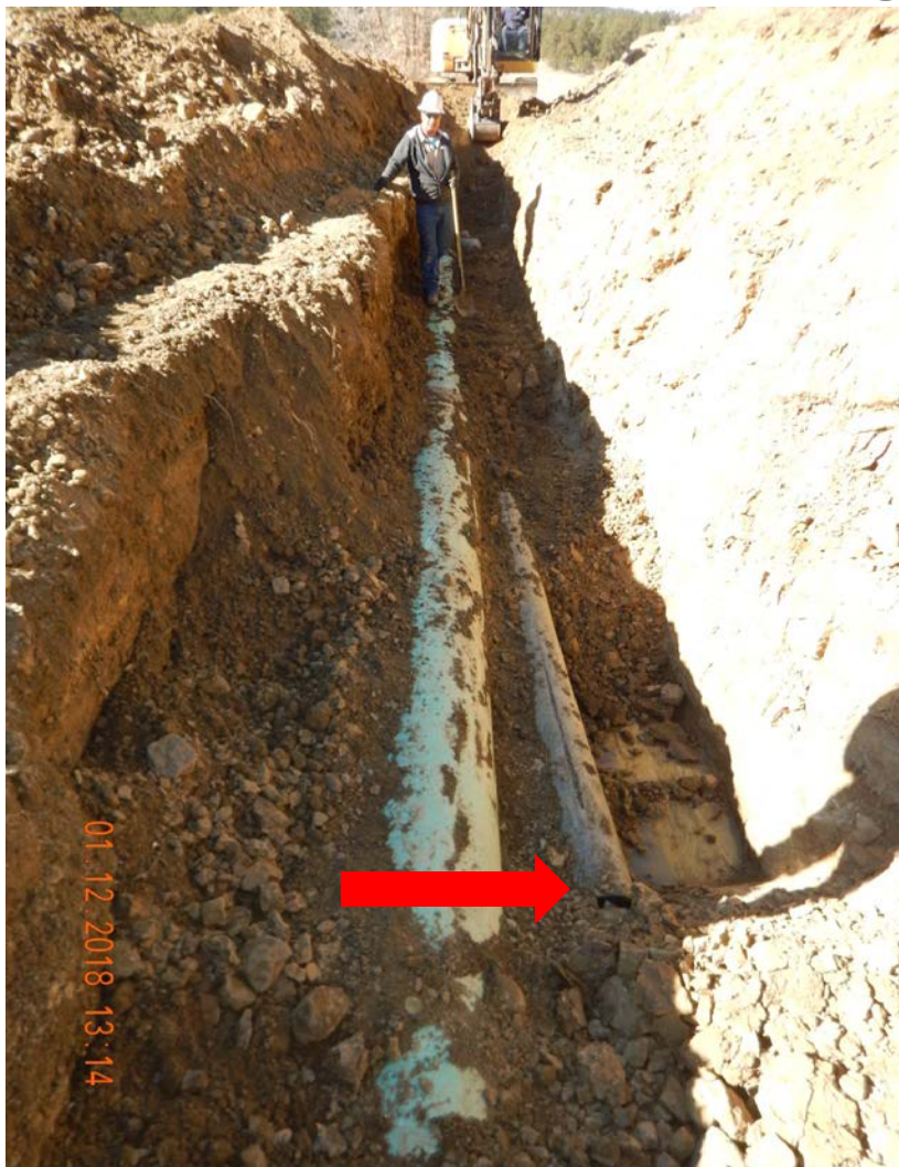
Produced water line break and excavation.
