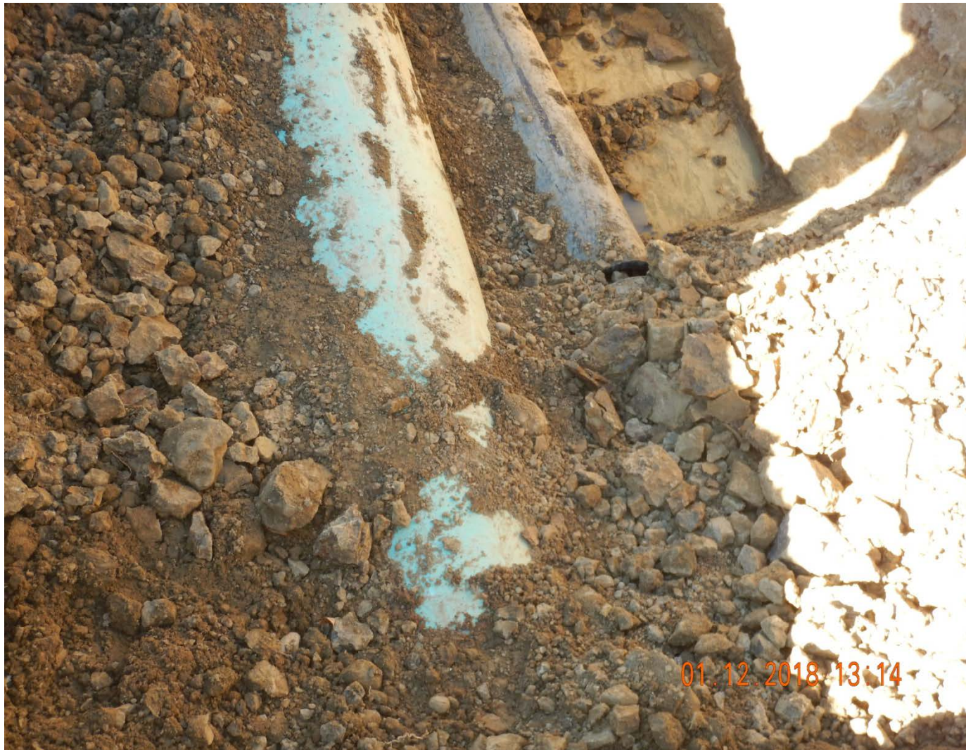
Produced water line break
