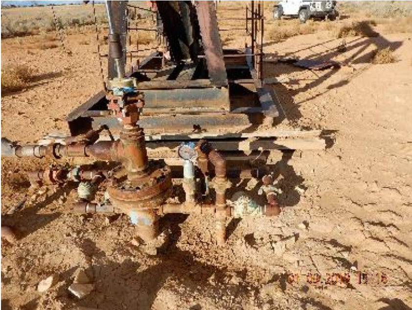
Photo 3: Wellhead flowlines right side.
