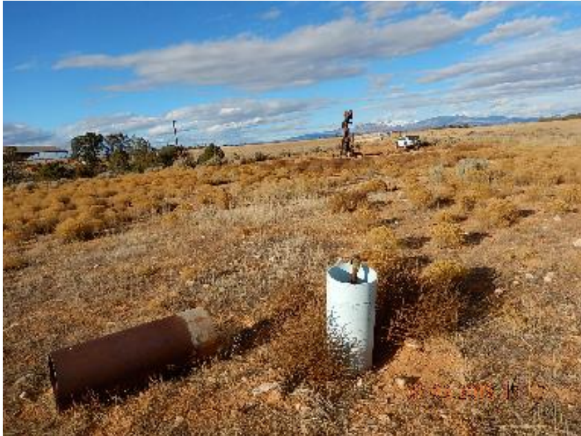
Photo 5: 1" steel riser with pump jack in background.
