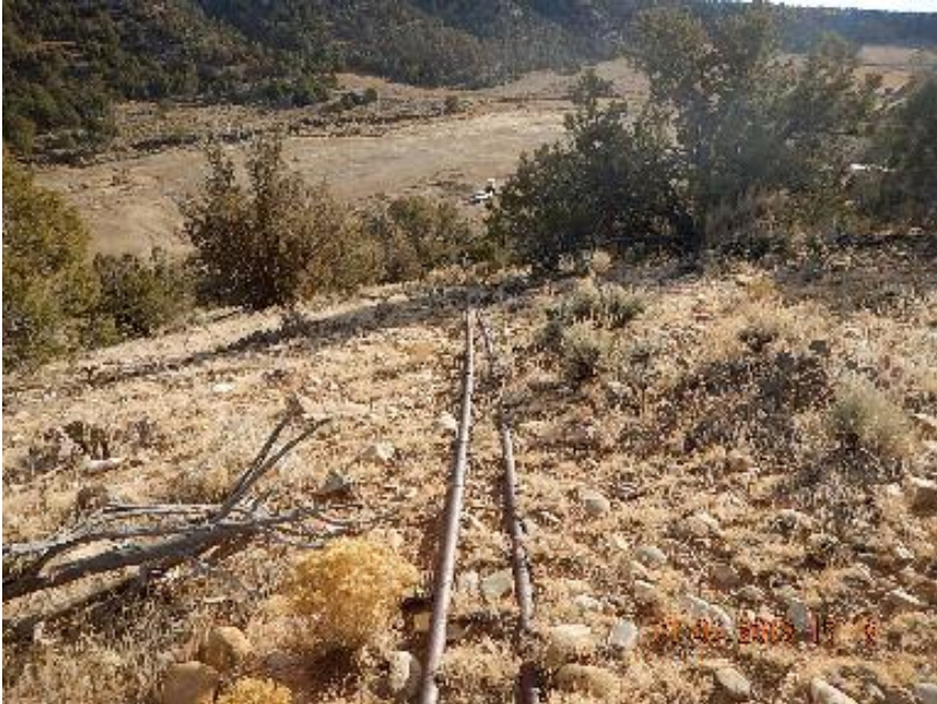
Photo 7: 3" steel lines heading down slope.
