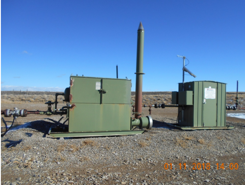
Separator and meter housing
