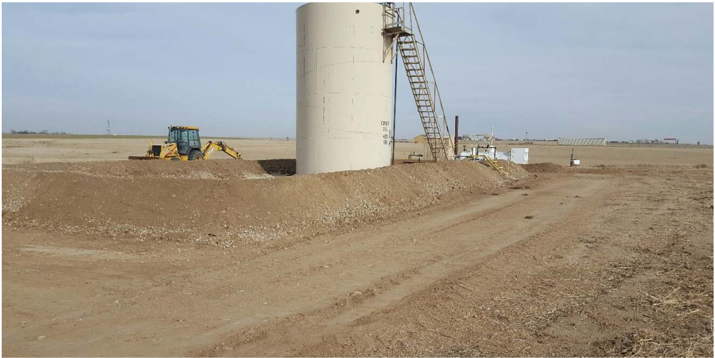
Figure #1 Berms have repaired
