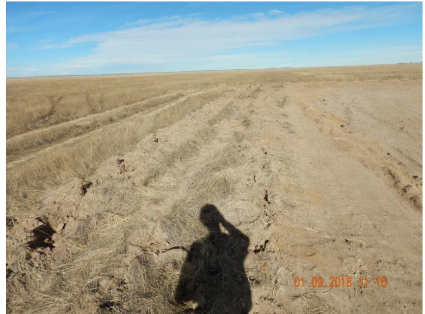
Photo 2. Photo taken from the western location, facing North. Operator has installed surface roughening BMP around the perimeter of the location which should be used in conjunction with other stormwater BMPs. Portions of the surface roughening BMP are in need of maintenance.
