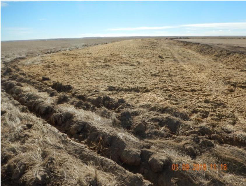
Photo 5. Photo taken from the northeast location, facing South. Appears the Operator has salvaged and stored topsoil along the eastern location. Topsoil has been temporarily stabilized with hydromulch.
