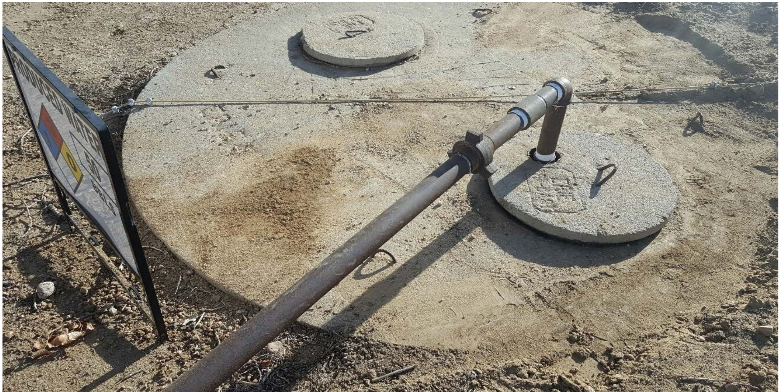
Figure #1 Damaged tank cover has replaced
