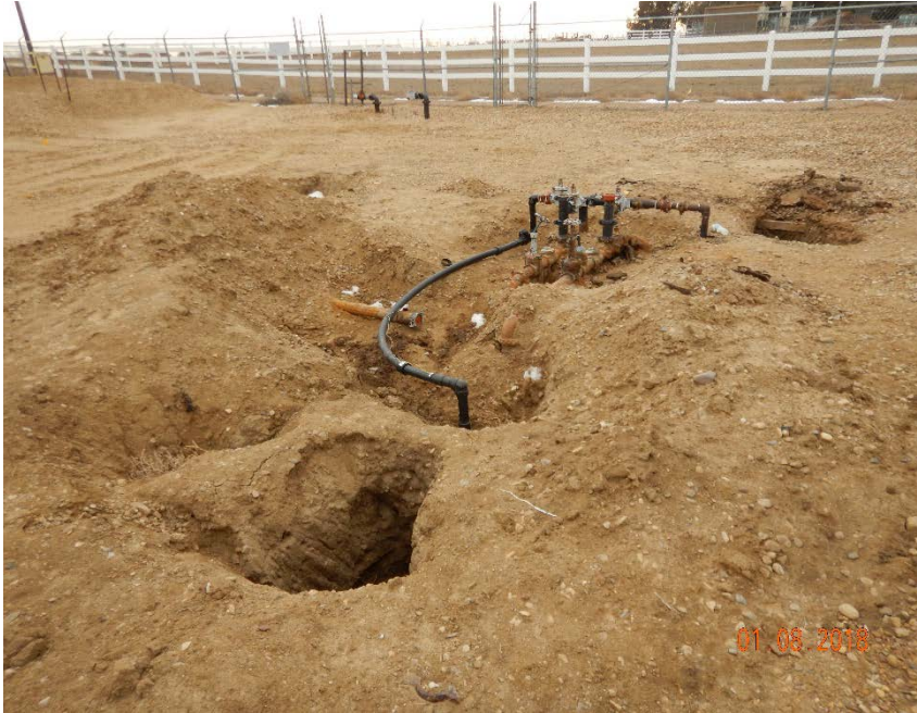
Photo #5 – View of partially-excavated flowline manifold from NW corner.
