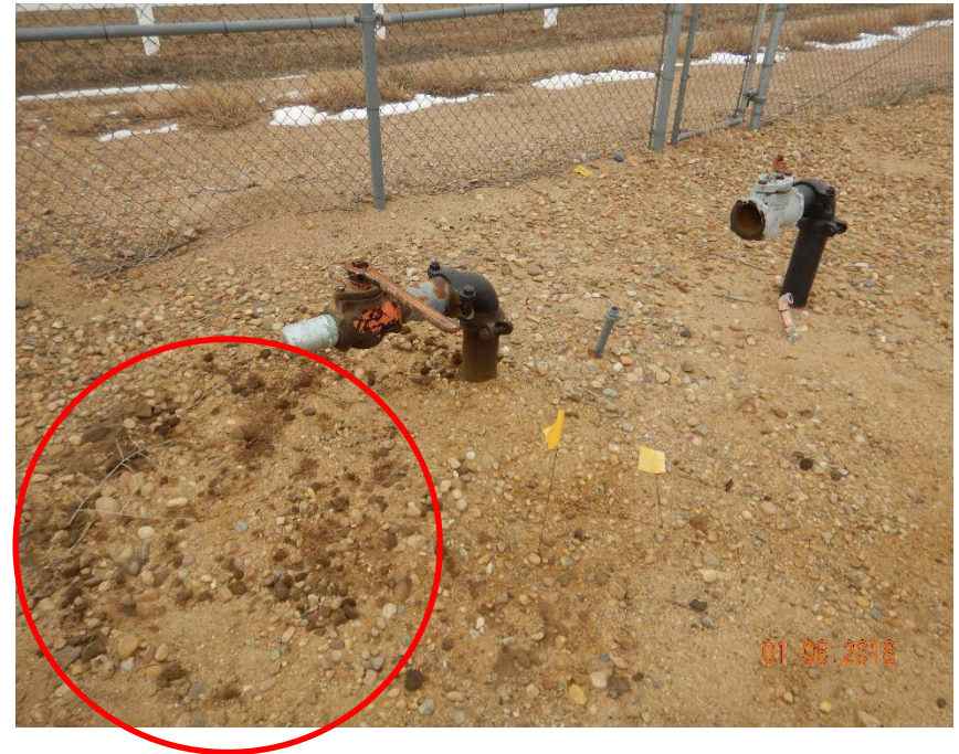
Photo #4 – Steel 4" flowline risers with 90-degree bend located SW of crude oil ASTs. Note localized accumulations of oily waste underlying riser with bullplug installed.
