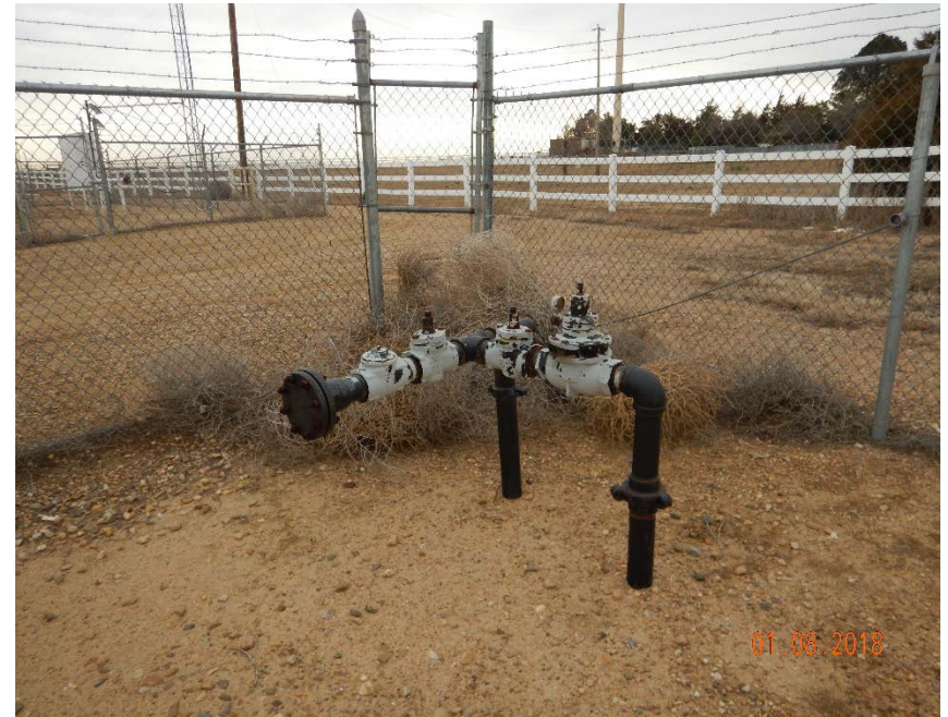
Photo #18 - Flowline risers located east of produced water vault (2).
