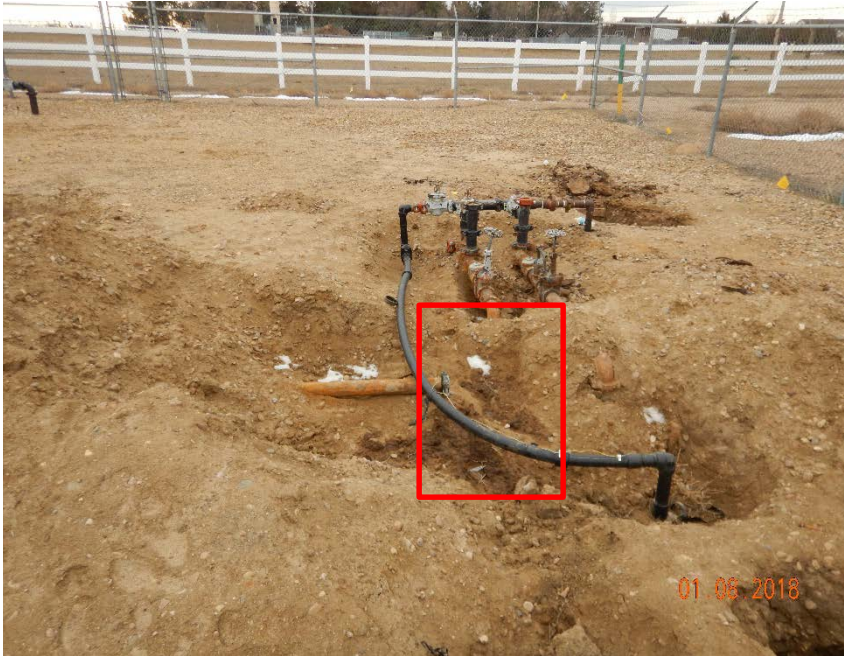
Photo #7 – Localized accumulations of oily waste beneath exposed flowline.
