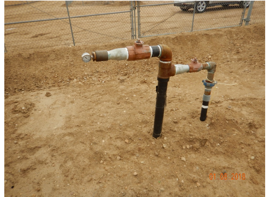
Photo #12 – Flowline risers located between horizontal separators.
