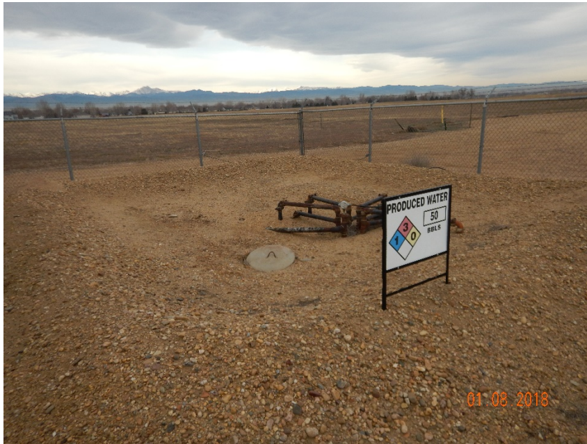
Photo #15 – Produced water vault on west side of facility with flowline risers.
