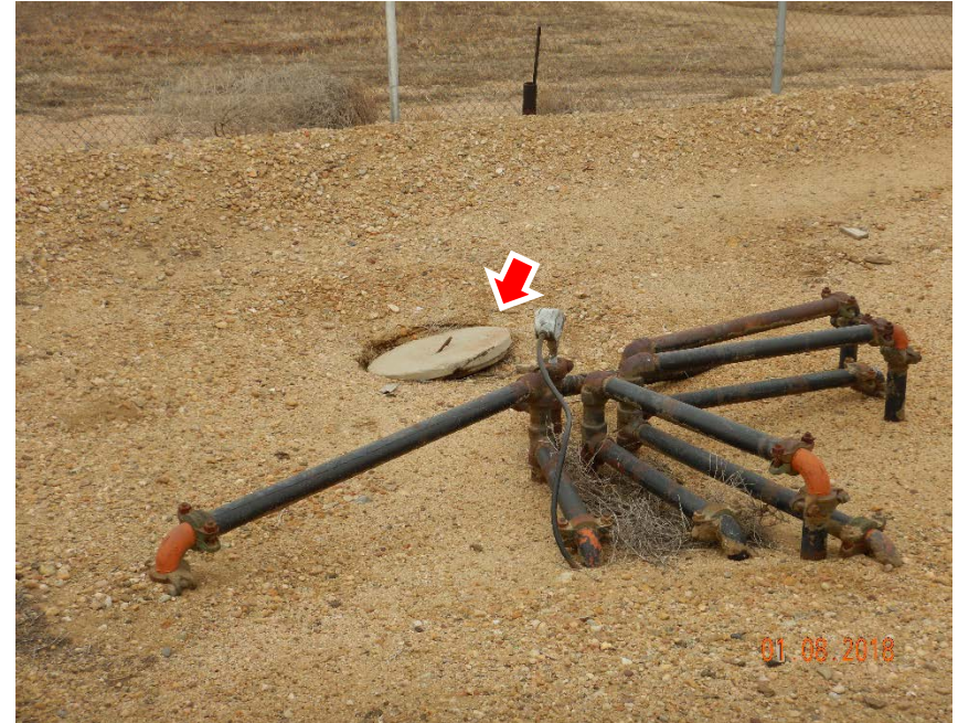
Photo #16 – Produced water vault cap/seal was improperly installed on inspection date.
