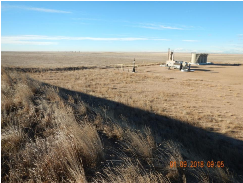
Photo 5. Photo taken from the eastern location on top of a stockpile, facing Southwest. Operator has failed to perform interim reclamation per Rule 1003.b. to reduce disturbance areas only reasonably needed for production operations.
