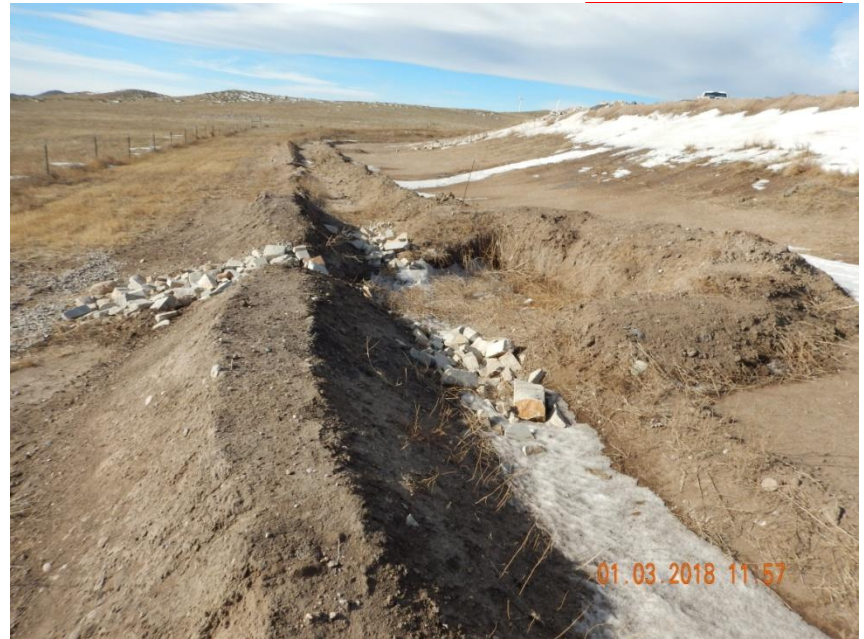
Photo 6. Photo taken from the western sediment trap, facing West. Appears the Operator has made improvements to the sediment trap (enlarged the depth and improved the embankment berms). Inlet protection to the sediment trap has not been installed to good engineering practices. Appears the outfall of the sediment trap is higher than the ditches; therefore, the sediment trap would not properly function.
