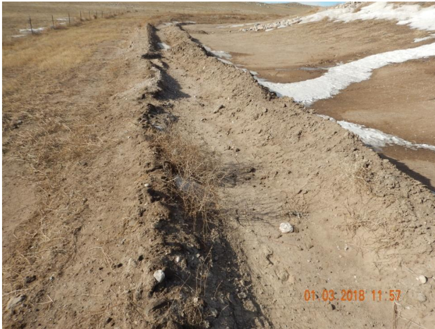
Photo 5. Photo taken from the southwestern location, facing West. Operator has not constructed the ditch and berm BMP with good engineering practices. Ditch BMP in need of maintenance.
