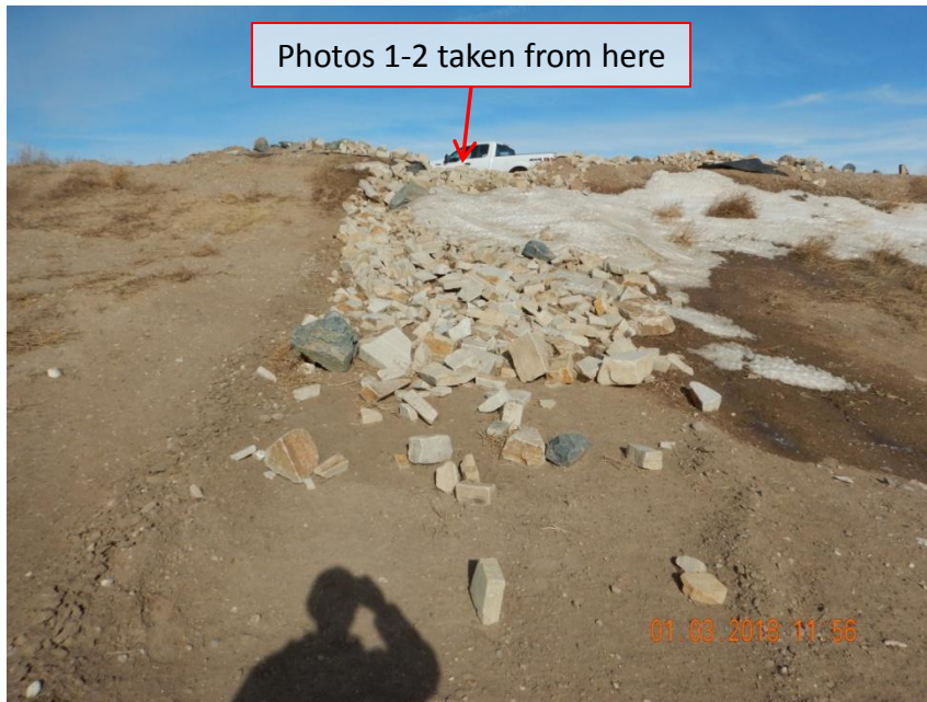
Photo 3. Photo taken from the southwestern location, facing North. Operator has haphazardly installed rock material that appears to be used as a berm BMP and a stabilized outfall to the lower perimeter ditch and berm BMP.
