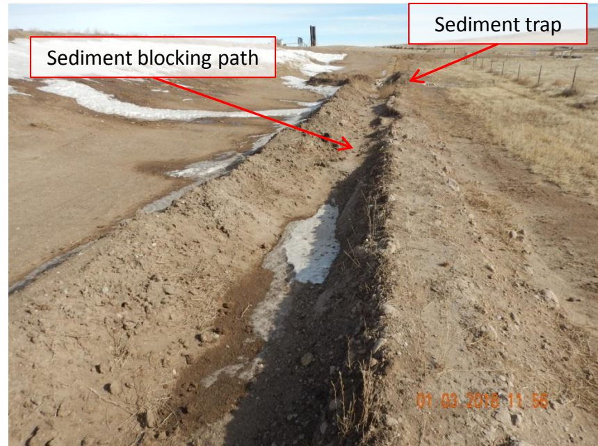
Photo 4. Photo taken from the southwestern location, facing East. Operator has constructed a ditch and berm BMP; however, there is sediment blocking the path that will not allow stormwater flows to travel to the sediment trap. Ditch BMP in need of maintenance.
