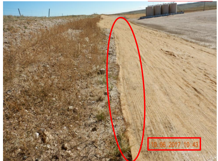
Photo 11. Photo taken from the northern cut slope area, facing East on October 6, 2017. Photo illustrates the Operator has not addressed the issue to properly install the erosion blanket.
