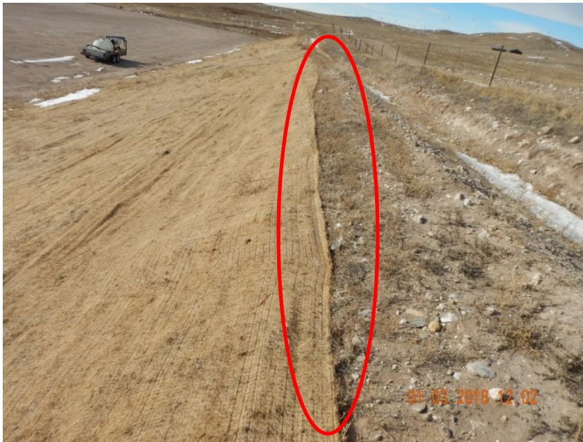
Photo 10. Photo taken from the northern cut slope area, facing West on January 3, 2018. Operator has not properly installed the erosion blanket using good engineering practices and has not addressed the issue since the previous inspection. Operator has not properly trenched and anchored BMP. Operator has not installed the BMP with good contact with the ground to avoid tenting.
