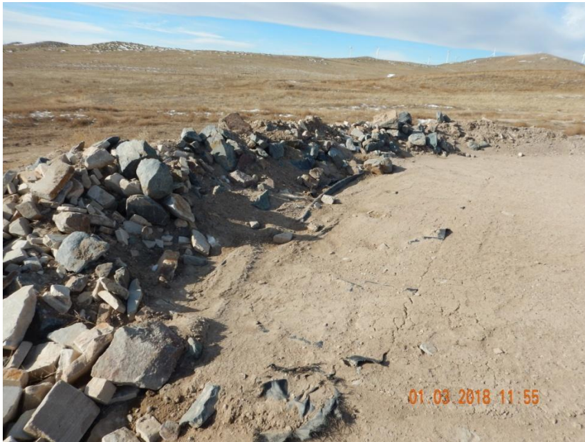
Photo 1. Photo taken from the southwestern location, facing West. Operator has not constructed the berm BMP with good engineering practices per Rule 1002.f.(2)., nor has the Operator repaired the berm BMP from the previous corrective action inspection.
