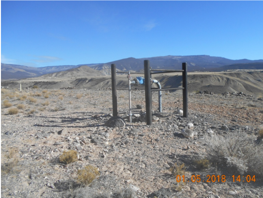
Flowline riser marked locked out/ tagged out
