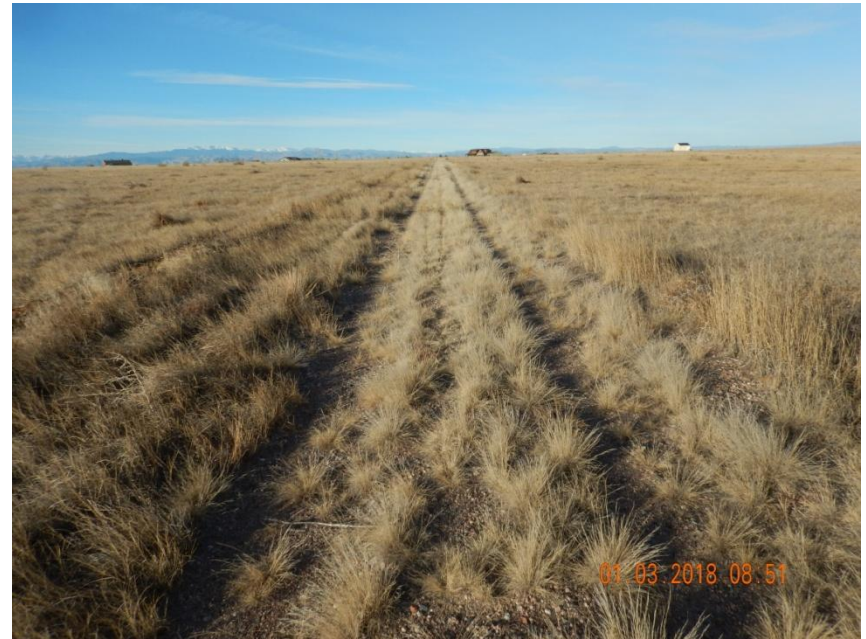
Photo 6. Photo taken from a portion of the access road, facing West. Gravel remains on access road and access road has not been contoured to match the surrounding landscape per Rule 1004 standards.
