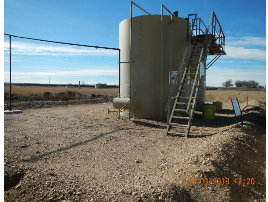
Erosion of berms at tank battery
