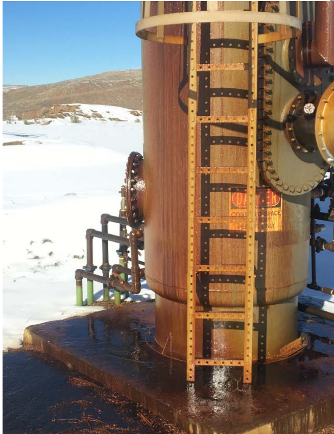
Photo taken 12/28/2017. Oil on ground around treater, it appears to be a greater amount of fluid than observed on 11/15/2017
