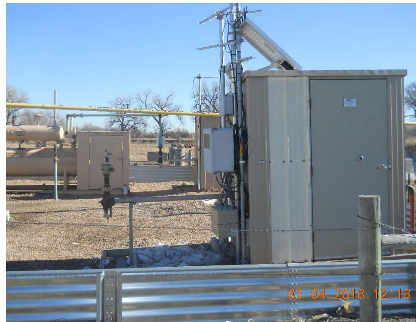
Unused/disconnected gas meter run
