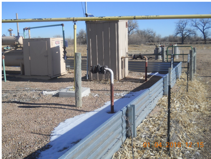
2" steel marked/unused riser
