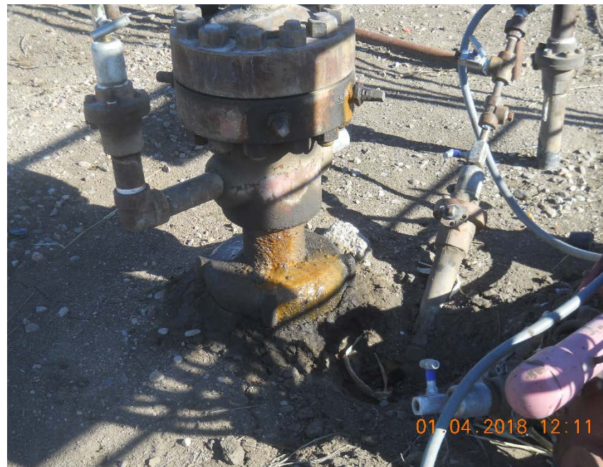
Wellhead is leaking/had leaked. Stained soil around wellhead
