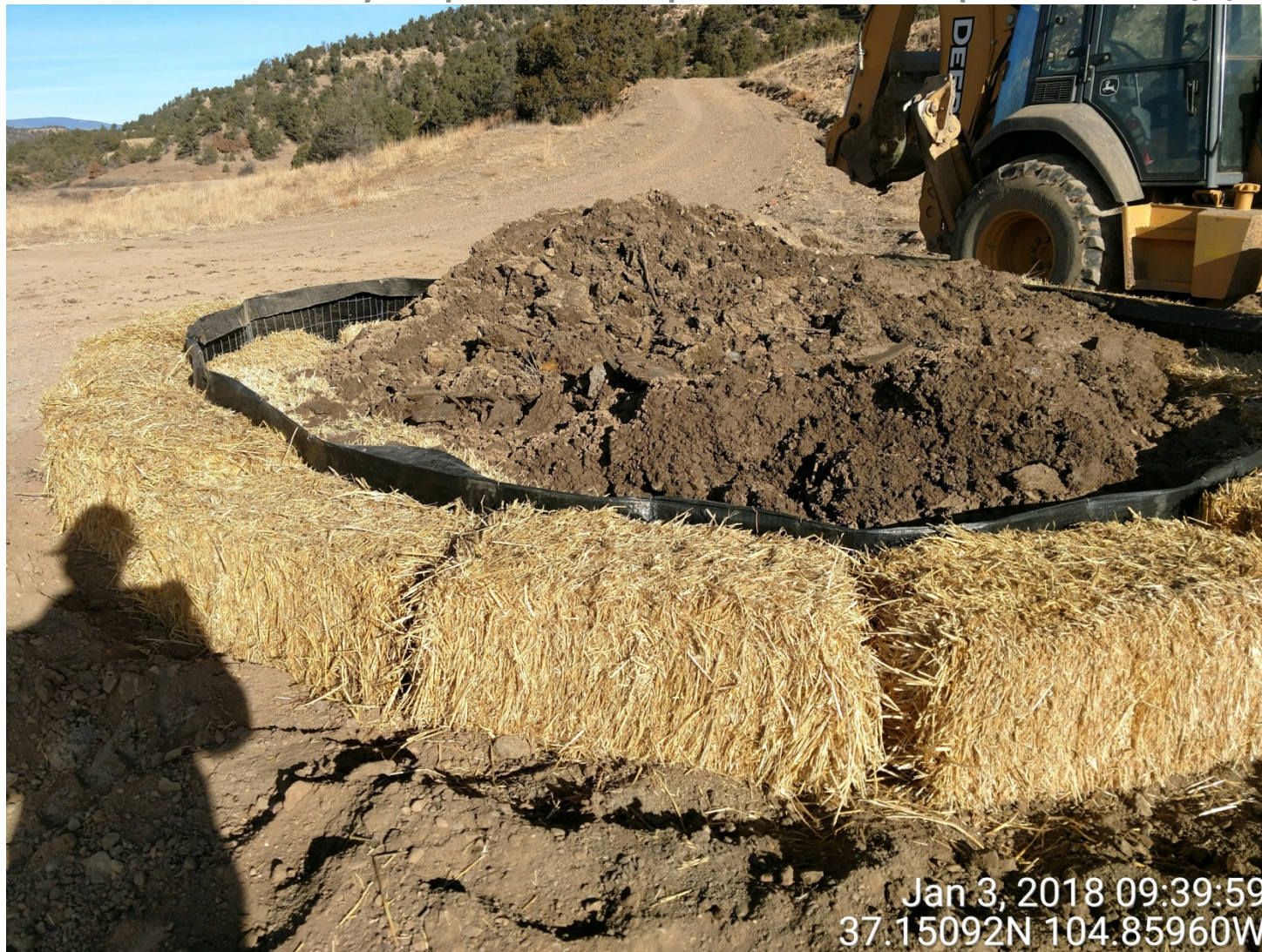
Impacted soil stored in secondary containment on well pad.
