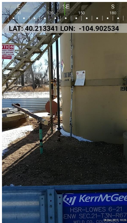
Photo 4 Flood anchoring on crude oil tank.
