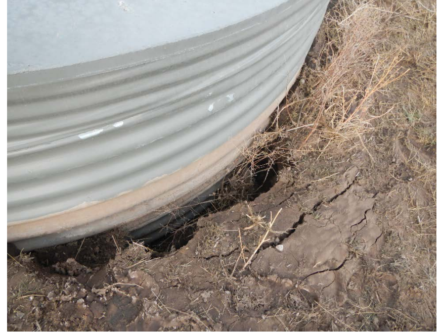
Spill erosion around valve can
