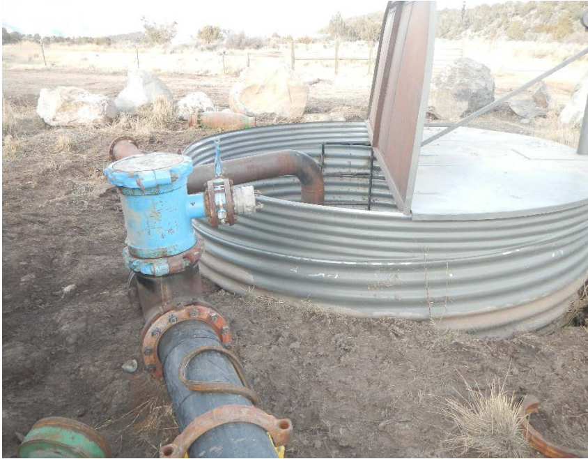
Pig receiver at valve can looking north
