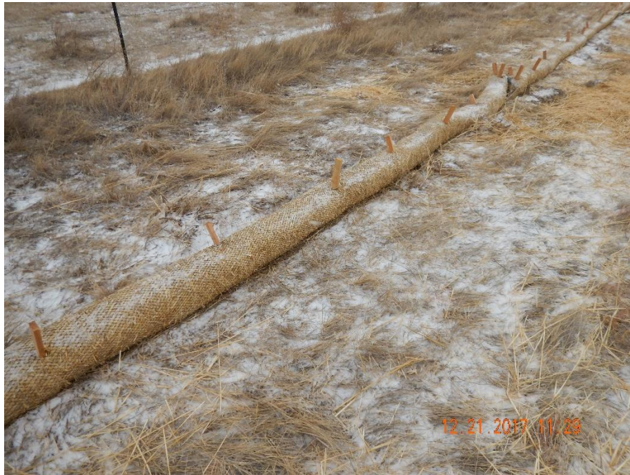
Photo 3: Photo of straw wattle used as a stormwater ponding BMP along the eastern perimeter of the location. Photo shows that wattle does not appear to have been installed with good engineering practices. Wattle does not appear to be sufficiently trenched and back-filled
