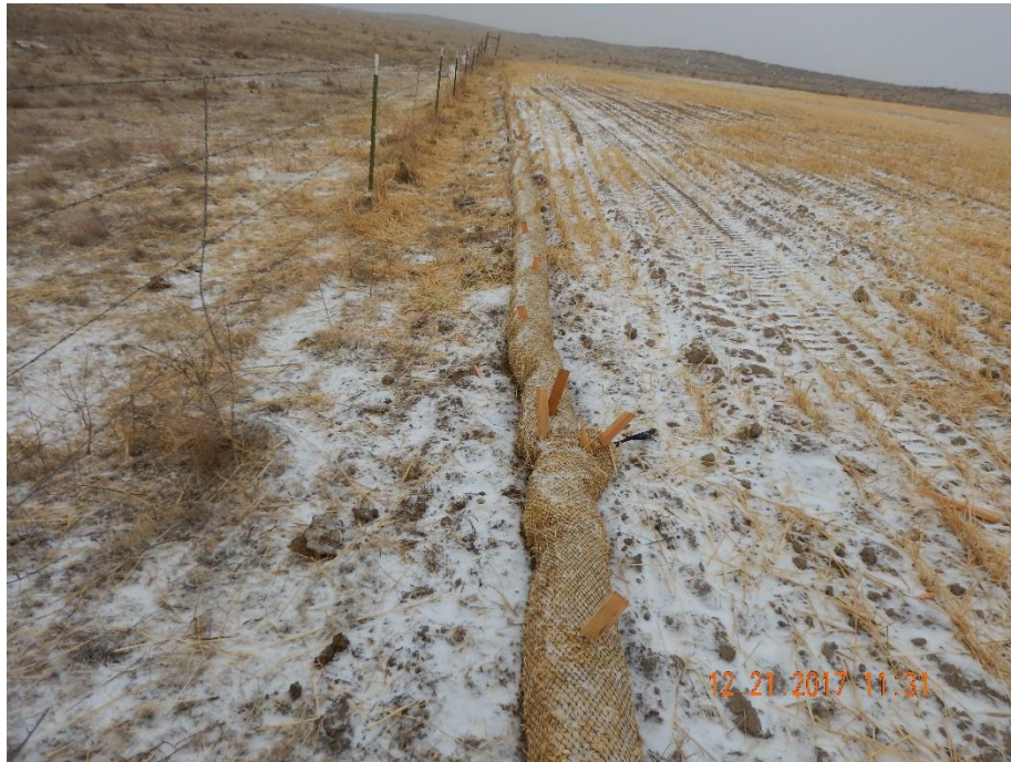
Photo 5: Photo of straw wattle used as a stormwater ponding BMP along the western perimeter of the location. Photo shows that wattle does not appear to have been installed with good engineering practices. Wattle does not appear to be sufficiently trenched and back-filled
