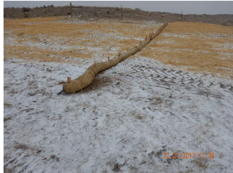
Photo 15: Photo of straw wattle BMP at the access road. Photo shows that wattle does not appear to have been installed with good engineering practices. Wattle does not appear to be sufficiently trenched and back-filled
