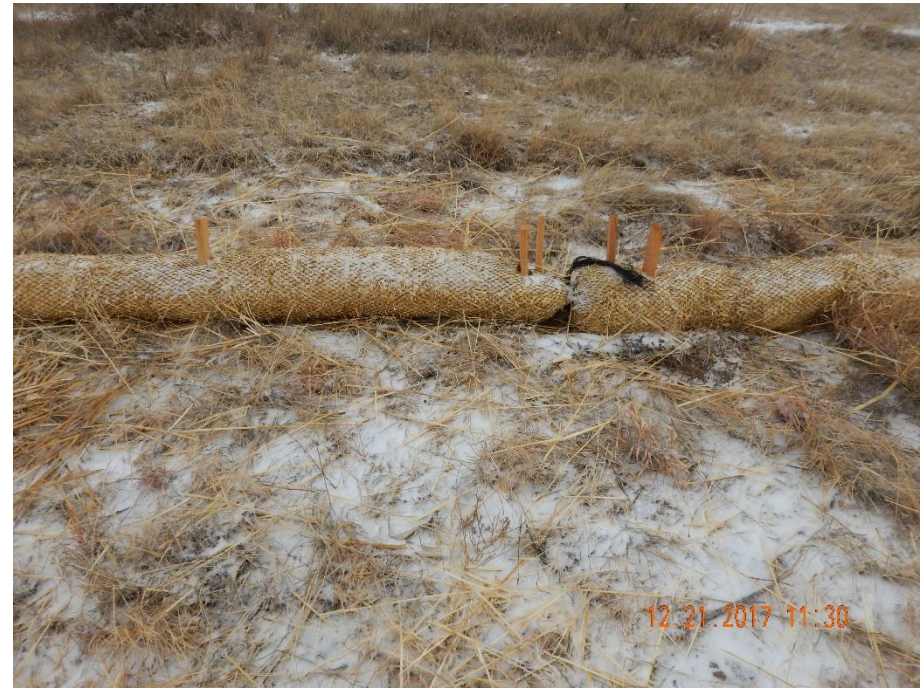
Photo 4: Photo of straw wattle used as a stormwater ponding BMP along the eastern perimeter of the location. Photo shows that wattle does not appear to have been installed with good engineering practices. Wattle does not appear to be sufficiently trenched and back-filled
