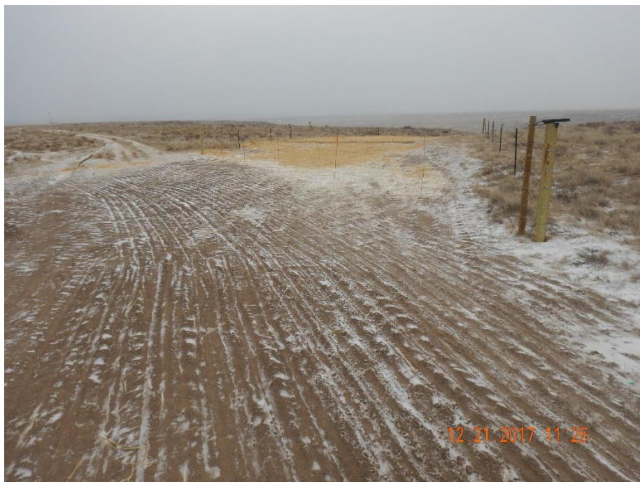
Photo 16: Photo taken from access road, northeast of the location. Photo at point where access road turns to the northwest. Photo shows operator appears to have only reclaimed a portion of the access road, leaving ~1/2 mile un reclaimed.
