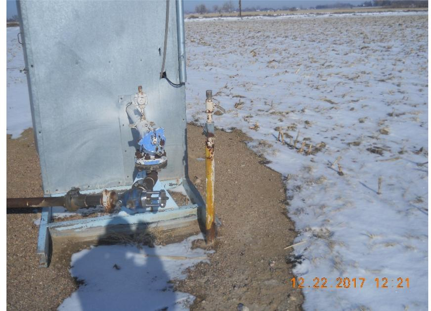
**2" steel unused/unmarked riser south of gas meter run**
