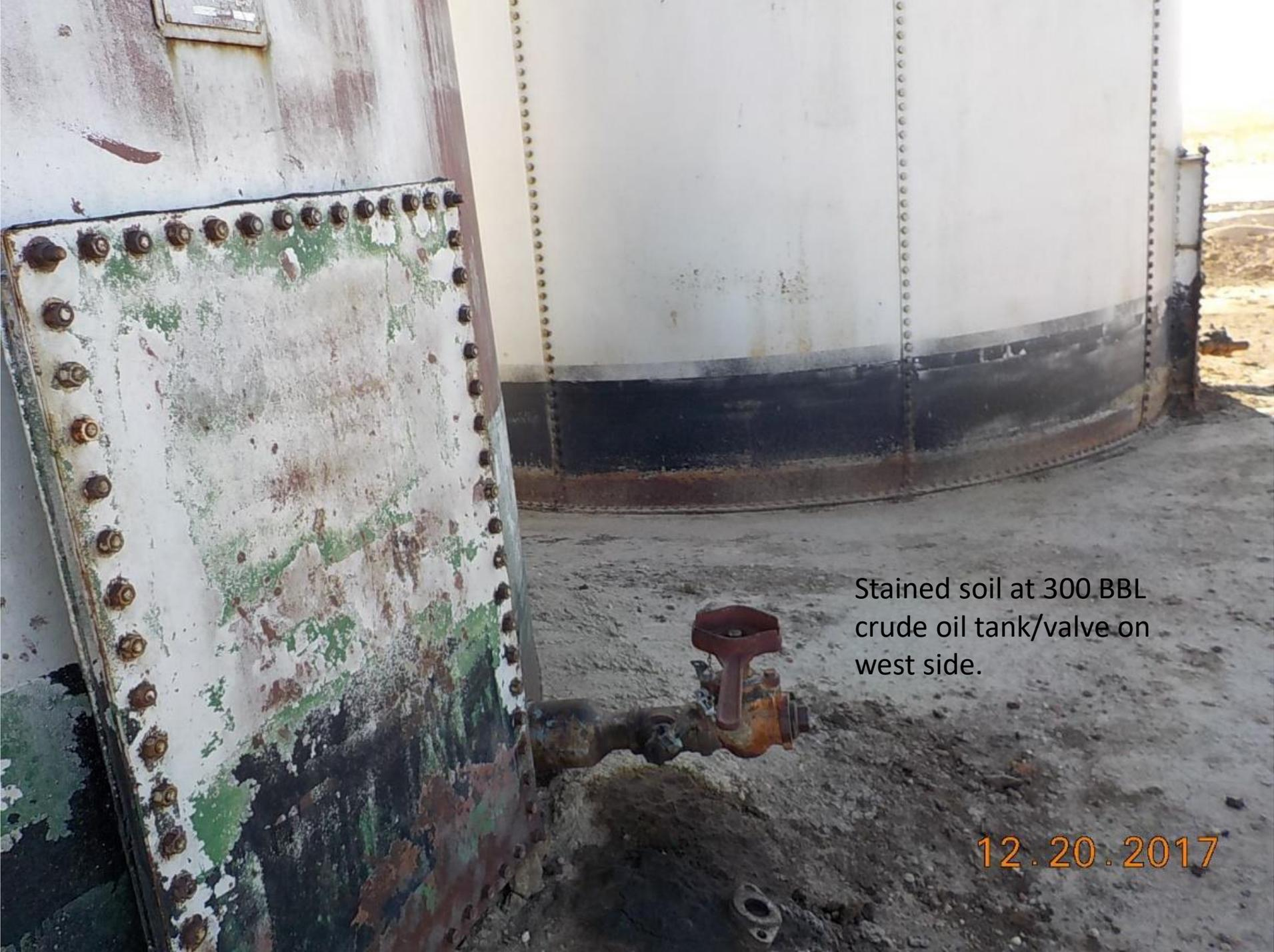
Stained soil at 300 BBL crude oil tank/valve on west side.
