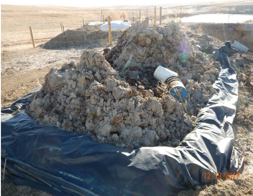
Photo #15 – View of NW lined stockpile of oily waste and debris. Note fenced skim tank with earthen berm in background.
