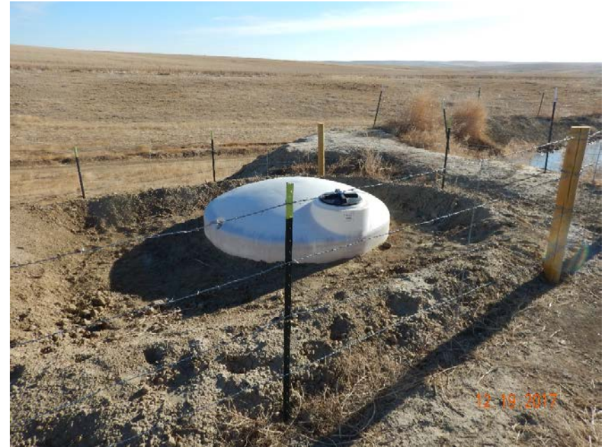
Photo #16 – View of skim tank from west. Tank lacked required volume/content labels and NFPA placard on inspection date.
