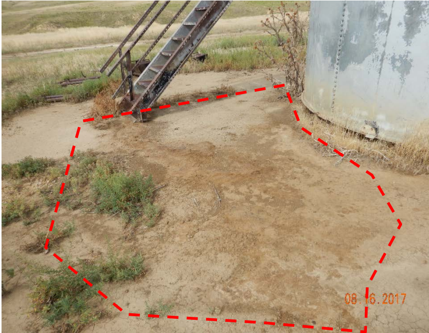
Photo #9 – Photo from AUGUST 16, 2017 illustrates historical accumulation of oily waste underlying area south of modular steel ASTs, which were removed prior to 12/19/2017 FIR. No visual evidence remains of these impacts as of 12/19/2017.
