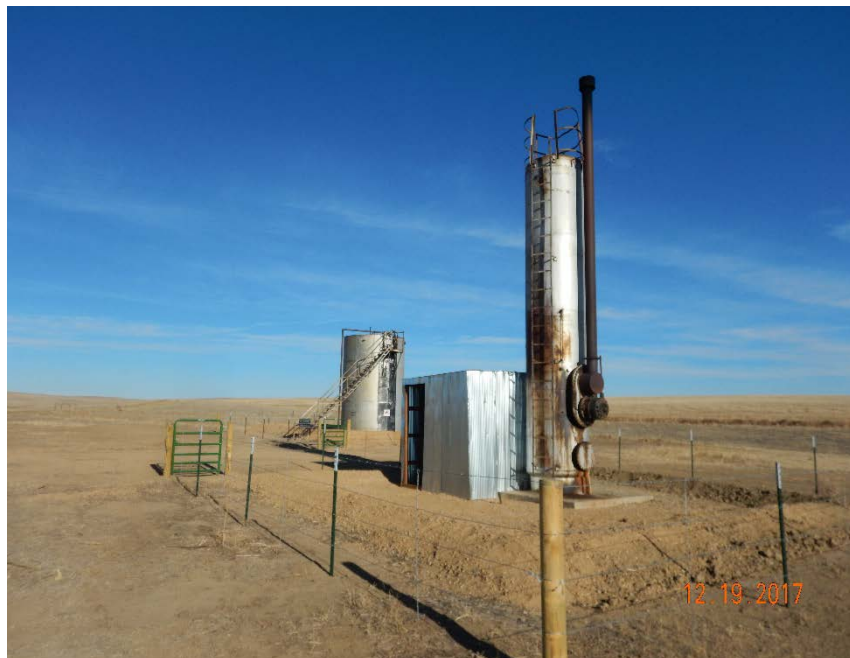
Photo #11 – View of vertical heater treater (VHT) with recently-installed fence and shed from SW corner.
