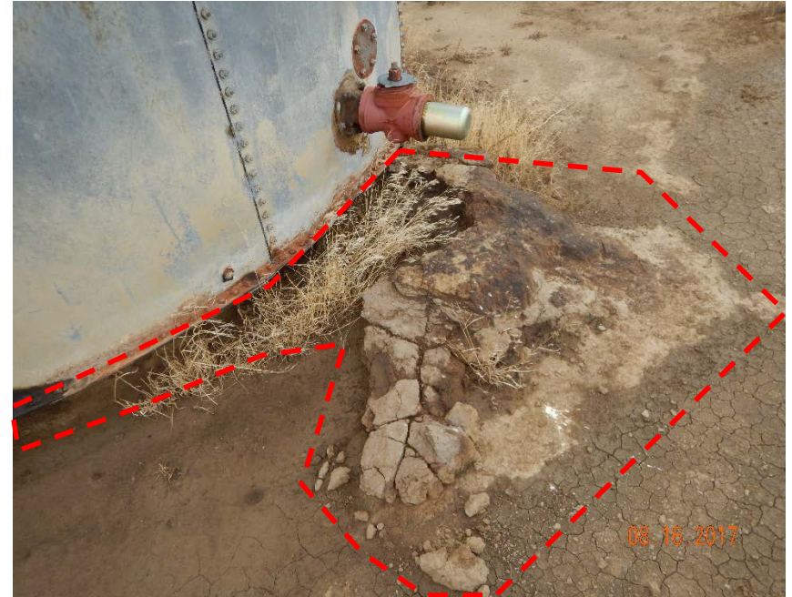
Photo #10 - Photo from AUGUST 16, 2017 illustrates historical accumulation of oily waste underlying modular steel ASTs, which were removed prior to 12/19/2017 FIR. No visual evidence remains of these impacts as of 12/19/2017.
