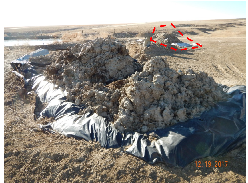
Photo #14 – Stockpiles of oily waste with debris located at NE and NW (background) corners of excavated skim pit. Note corrugated metal debris present inside of stockpiles and excavation.
