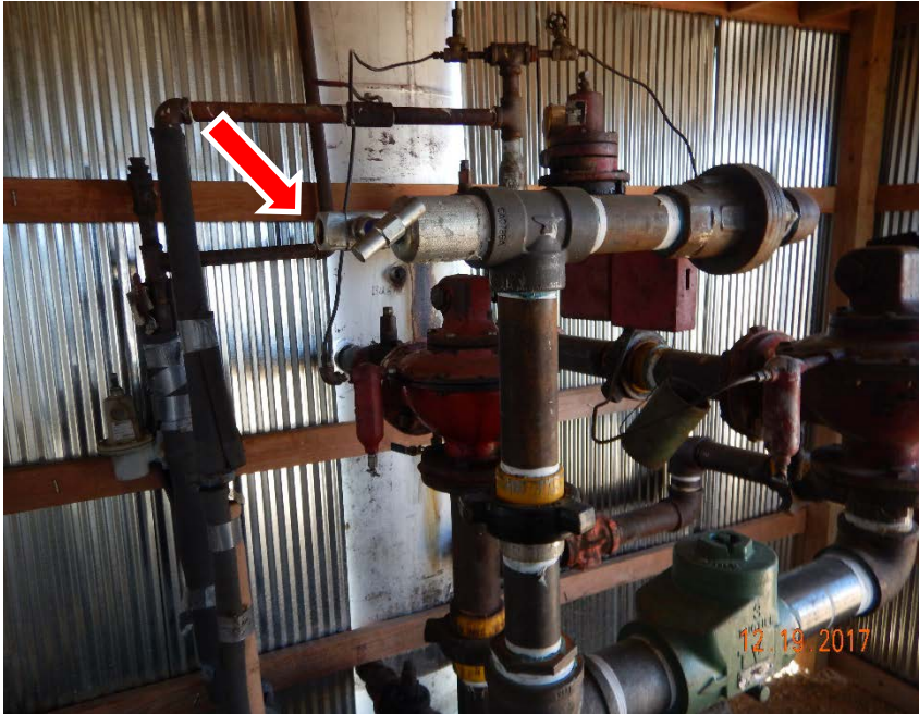
Photo #13 – View of valve that was most likely source of audible gas leak that was observed on inspection date. COGCC Inspector’s personal four-gas meter detected measurable concentrations of H_2S inside of VHT shed.
