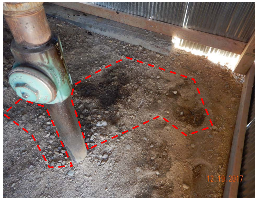
Photo #12 – Localized accumulation of oily waste inside of VHT shed.
