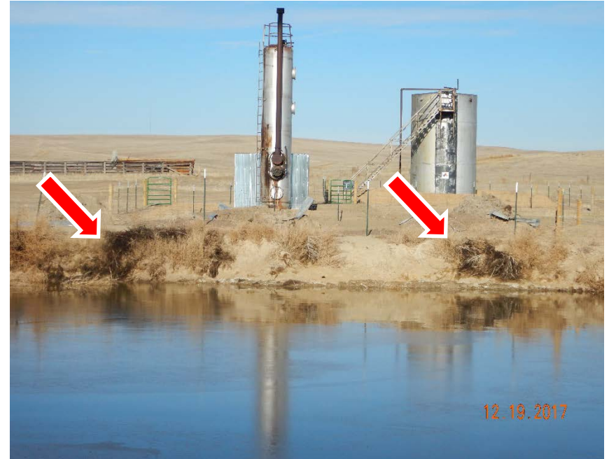
Photo #24 – View of oil-stained soil and vegetation inside of northern pit berm (from South).
