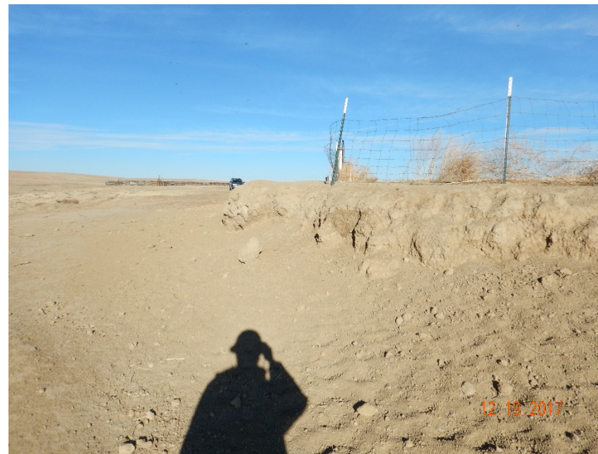
Photo #22 – View of eroded produced water pit berms, looking NW.
