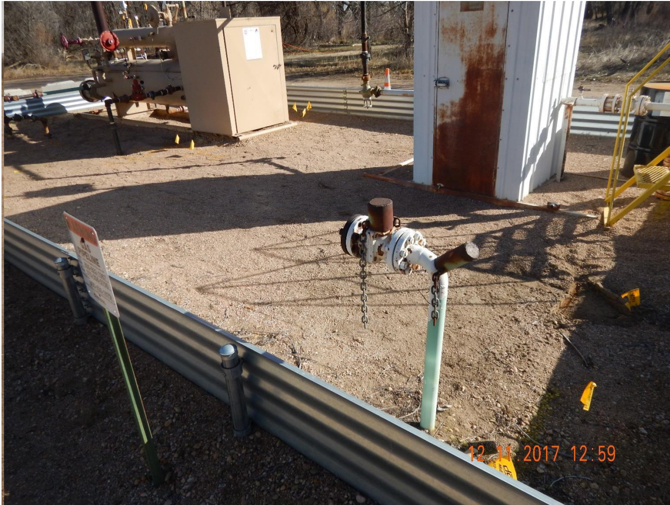
Photo 1: Photo taken from the eastern half of Extraction's Brantner Tank Battery Facility, facing southeast. Photo shows an abandoned pipe riser that has been identified as belonging to DCP. Riser requires removal in accordance to 1004.a.
