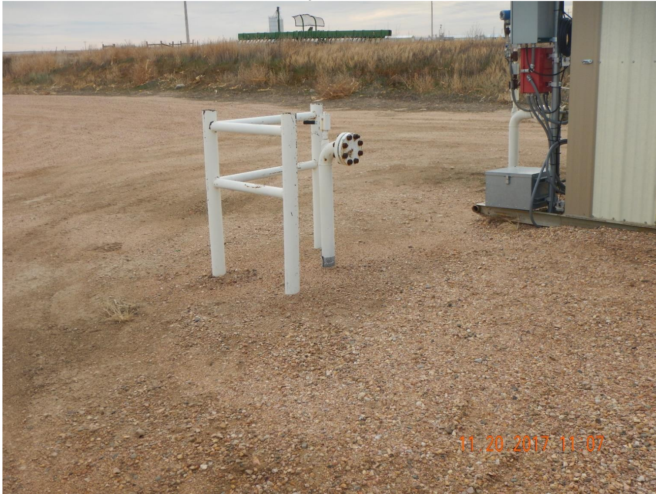
Photo 1: Photo taken from the western half of Noble's FOE A Tank Battery Facility. Photo shows an abandoned pipe riser that has been identified as belonging to DCP. Riser requires removal in accordance to 1004.a
