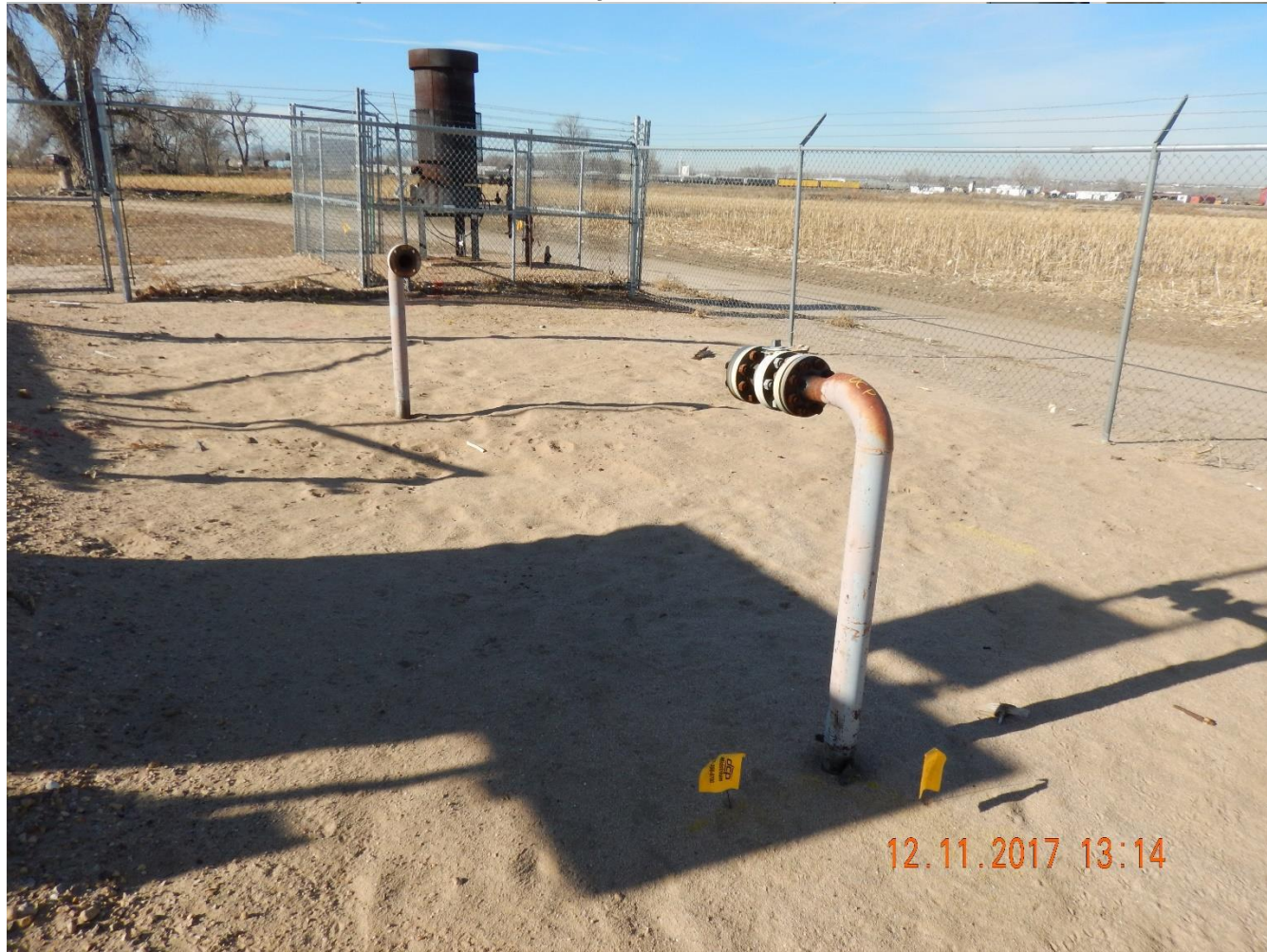
Photo 1: Photo taken from the western half of Noble's Stewart Tank Battery Facility, facing northwest. Photo shows two pipe riser that has been identified as belonging to DCP. Risers require removal in accordance to 1004.a
