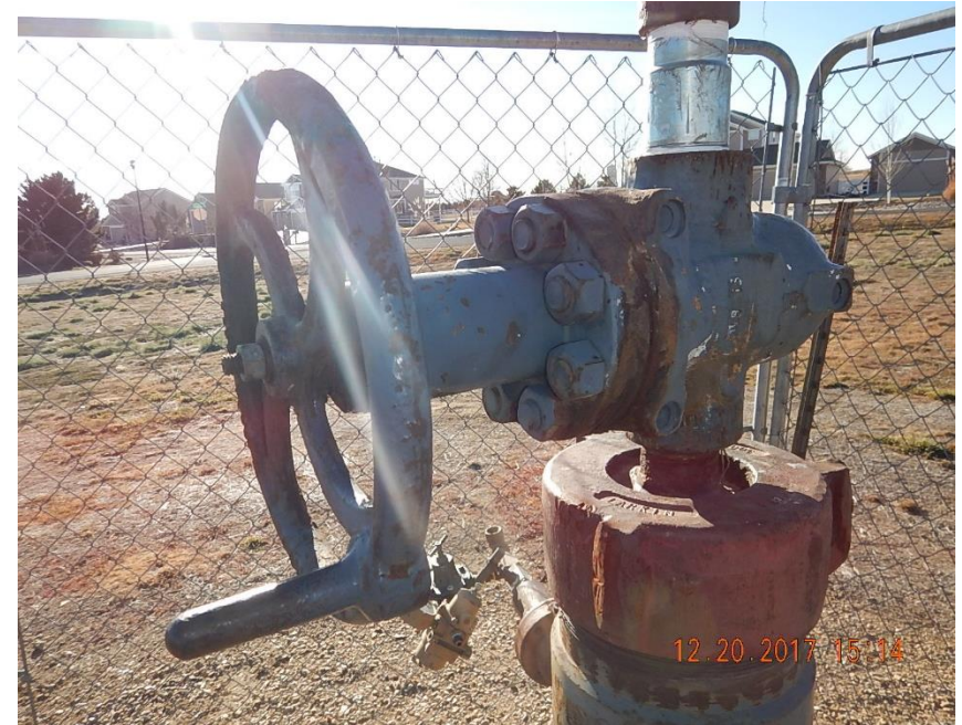
Master Valve – Leak identified at bolt up/ paint removed
