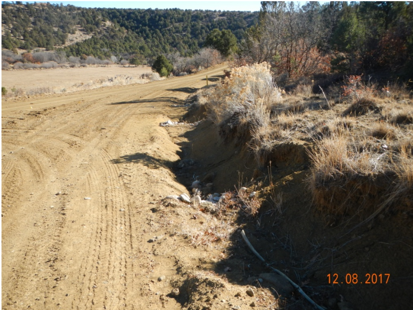
Photo 4. View of check dams along access that are full of sediment and need maintenance.
