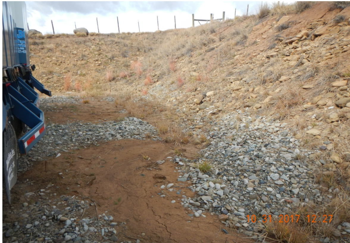
Photo 4 Migration of sediment onto pad surface.
