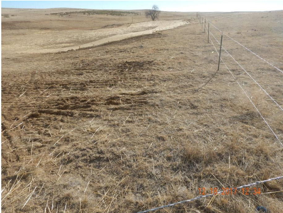
Photo 1: Photo taken from the west end of the location, facing southeast. Photo shows western slope of the well pad location has been recontoured/regraded and stabilized per the CA.
