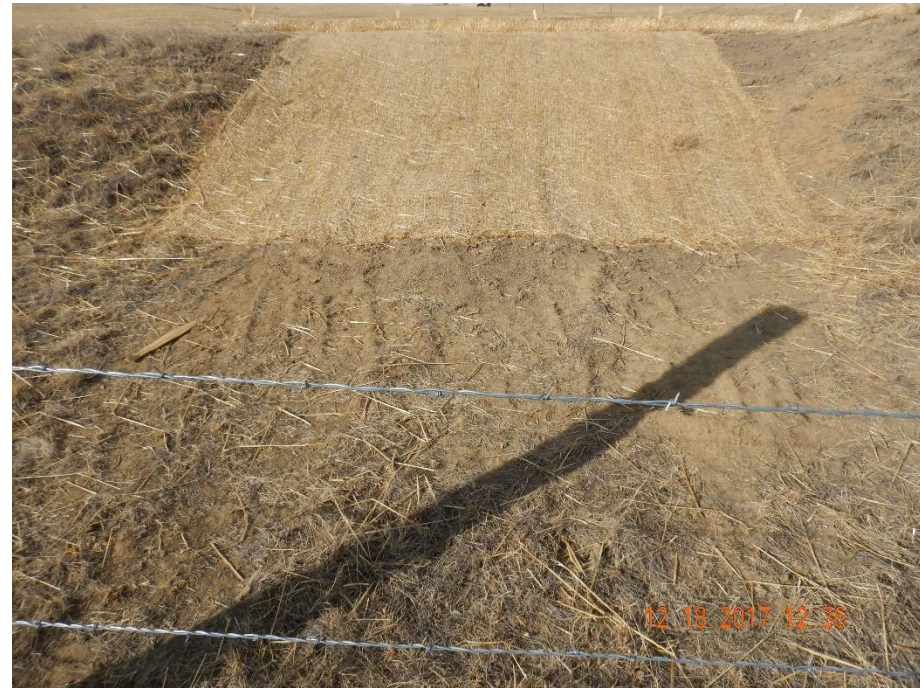
Photo 8: Photo taken from the southeast end of the location. Photo shows areas where erosion degradation was evident appear to have been repaired and stabilized.
