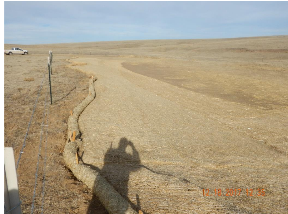
Photo 6: Photo taken southwest corner of the well location, facing north. Photo shows well pad appears to have been recontoured/regraded, seeded and stabilized w/ matting.
