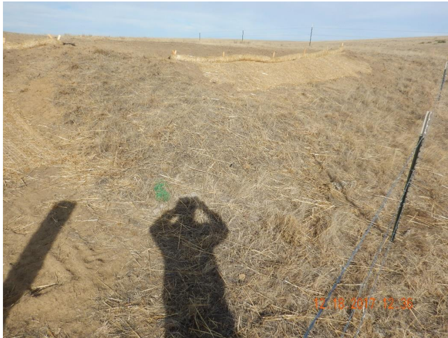
Photo 7: Photo taken from the southeast end of the location. Photo shows areas where erosion degradation was evident appear to have been repaired and stabilized.
