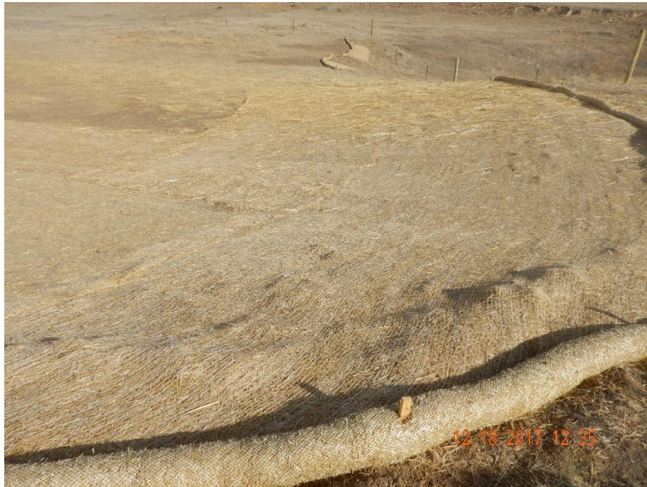
Photo 5: Photo taken southwest corner of the well location, facing east. Photo shows well pad appears to have been recontoured/regraded, seeded and stabilized w/ matting.
