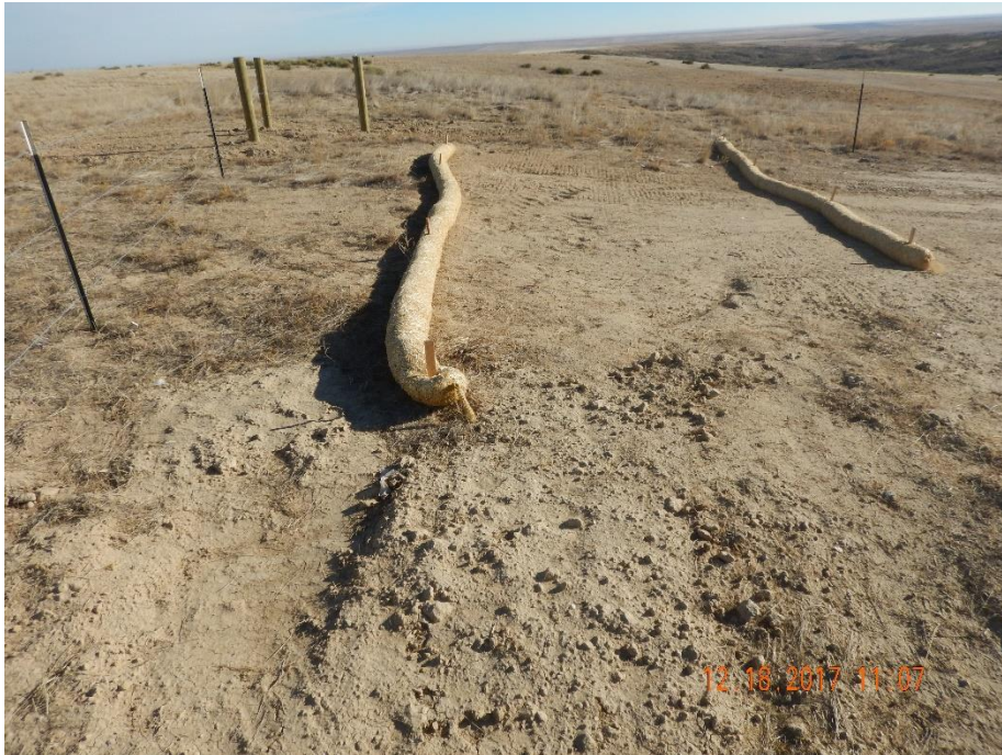
Photo 1: Photo taken from the northwest end of the fenced reclamation area (on slope), facing east. Photo shows straw wattles BMPs have not been installed in accordance to good engineering practices. Previous inspections required operator to perform reclamation and ensure erosion controls are implemented to stabilize the seeded soil. Photo shows the disturbance area appears to have been seeded (striations in soil suggest a no-till seed drill was used), however no erosion/stabilization controls appear to have been implemented to stabilize the seeded soil per the corrective action. This has allowed stormwater degradation to continue on the location.
