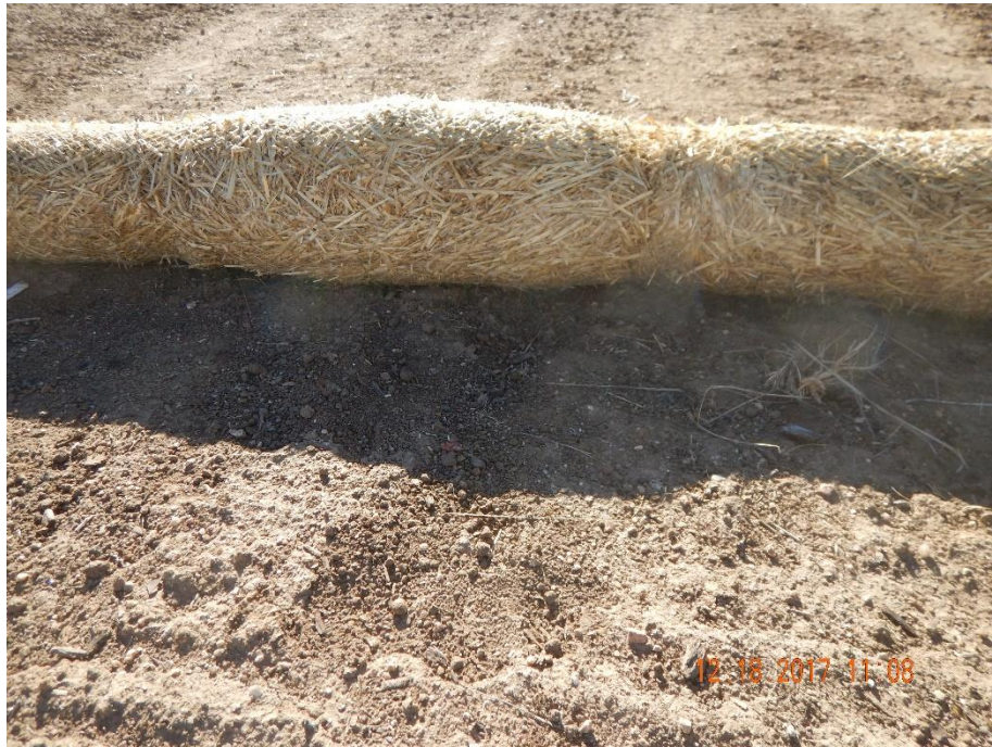
Photo 5: Photo shows straw wattles BMPs have not been installed in accordance to good engineering practices. Straw wattles are a stormwater ponding BMP that is required to be trenched below grade and backfilled in order to work in proper functioning condition.
