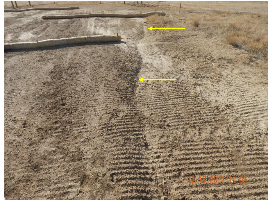
Photo 6: Photo taken from within the disturbance area on the slope, facing south. Photo shows that no erosion controls were implemented to stabilize the seeded soil, allowing erosion degradation to continue (yellow arrow).
