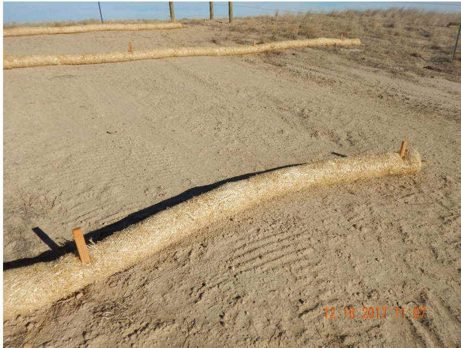
Photo 3: Photo taken from within the disturbance area on the slope, facing northeast. Photo shows straw wattles BMPs have not been installed in accordance to good engineering practices. Photo also shows the disturbance area appears to have been seeded (striations in soil suggest a no-till seed drill was used), however no erosion controls were implemented to stabilize the seeded soil per the corrective action.
