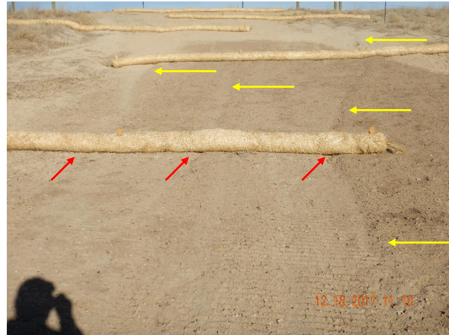
Photo 8: Photo taken from within the disturbance area on the slope, facing north. Photo shows that no erosion controls were implemented to stabilize the seeded soil, allowing erosion degradation to continue (yellow arrow). Photo also shows straw wattles BMPs have not been installed in accordance to good engineering practices, and stormwater has cut underneath the BMP (red arrow).
