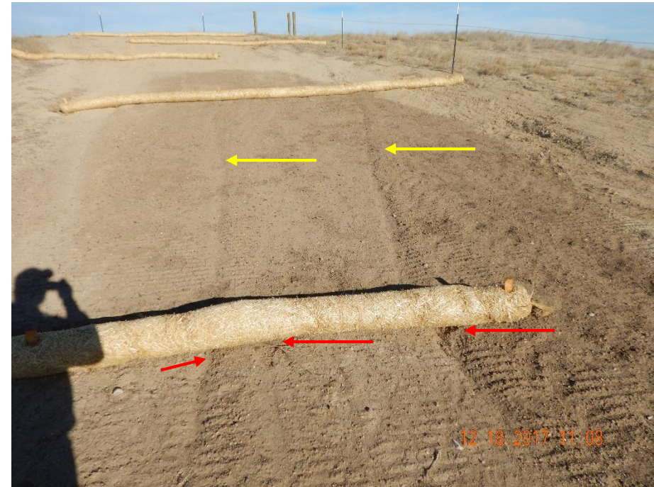
Photo 4: Photo taken from within the disturbance area on the slope, facing northeast. Photo shows that no erosion controls were implemented to stabilize the seeded soil, allowing erosion degradation to continue (yellow arrow). Photo also shows straw wattles BMPs have not been installed in accordance to good engineering practices, and stormwater has cut underneath the BMP (red arrow).
