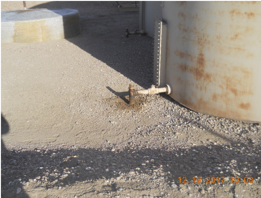
Stained soil at drain line on south crude oil tank
