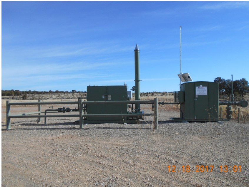
Separator and Meter housing with sign
