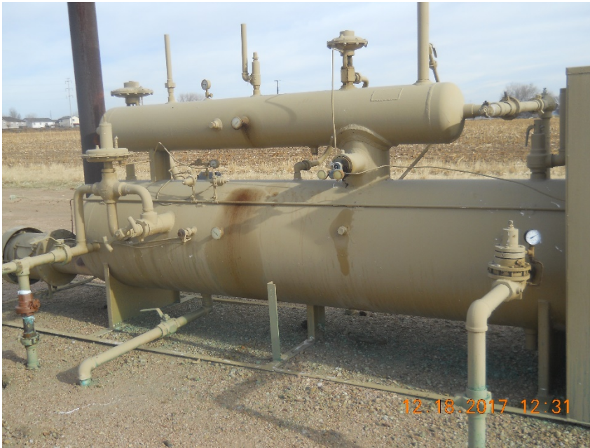
Leaking fittings on separator
