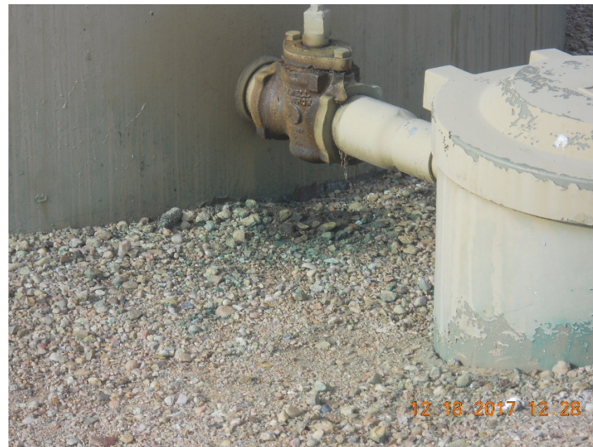
Stained soil under load line valve on crude oil tank
